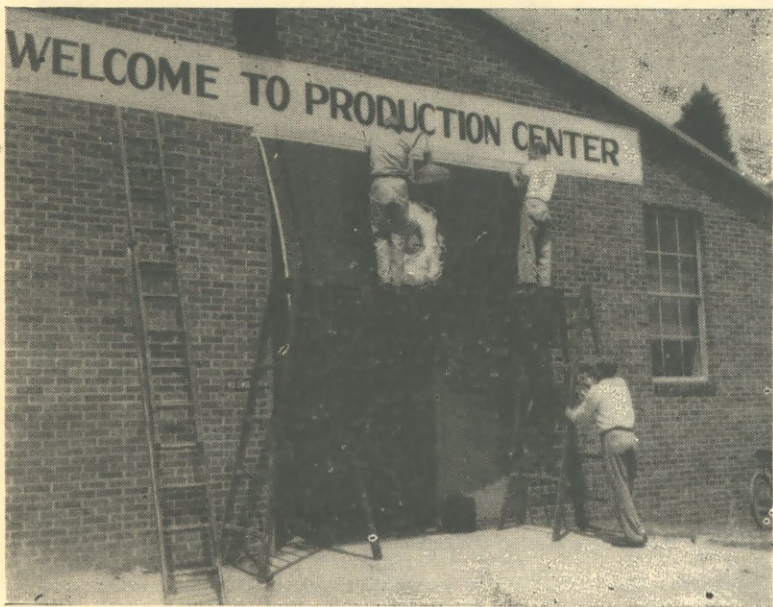
PREPARATIONS The Production Center is "dressed up" for the open house with a welcome banner and the bright red Colonial Williamsburg house flag.
