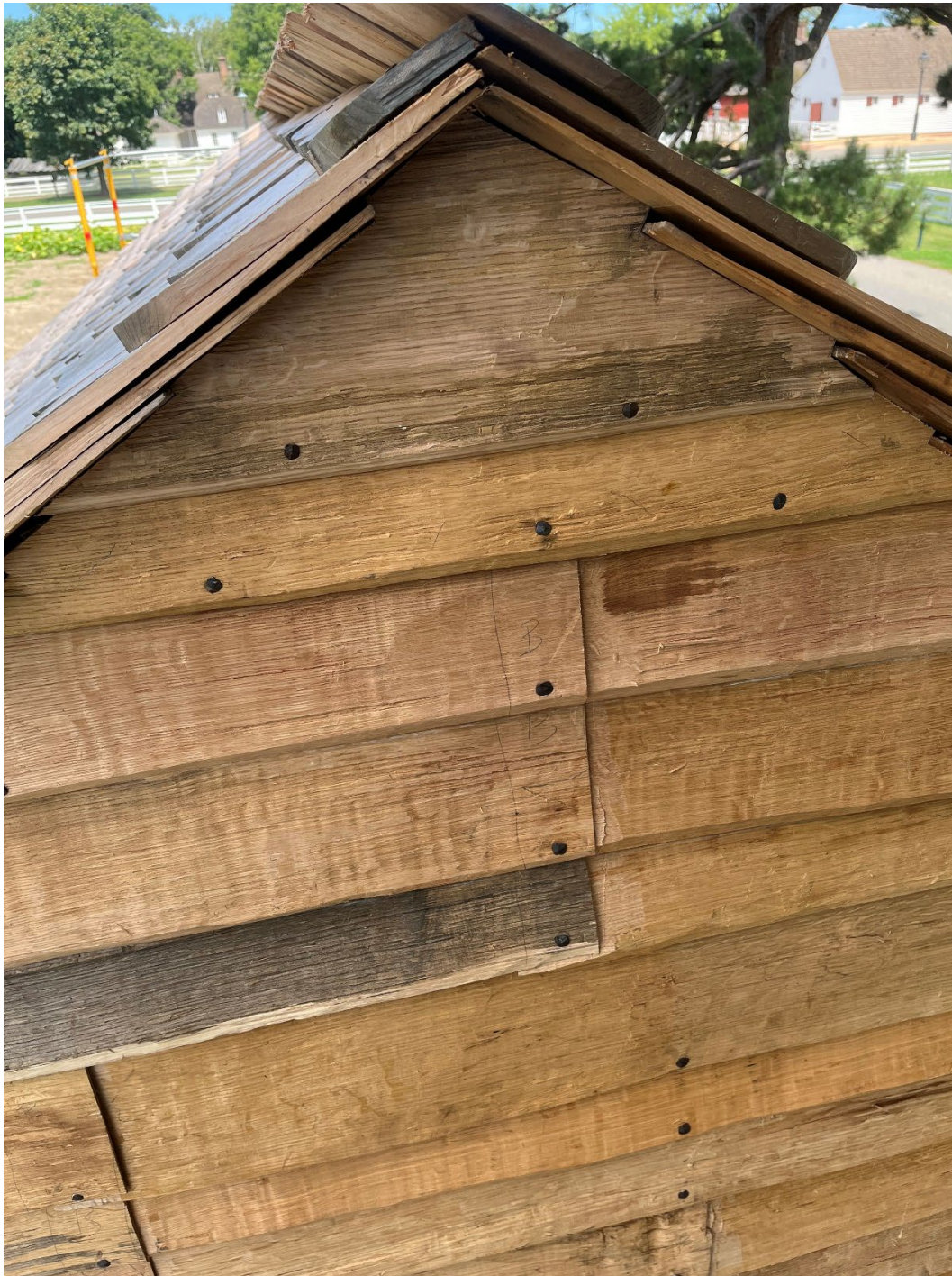
Clapboards installed on wagon shed.
