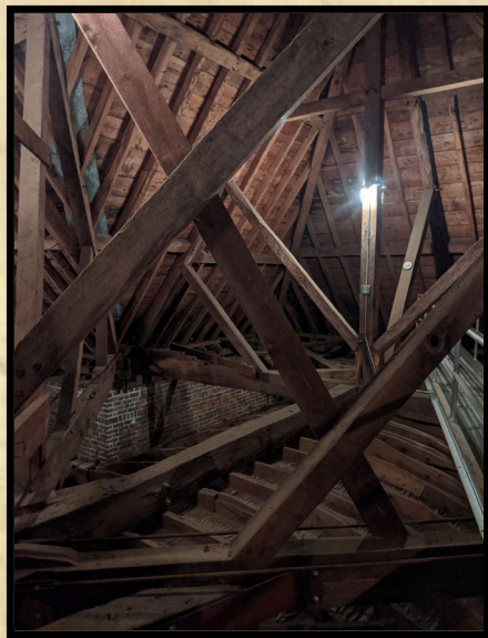
The attic at Christ Church
