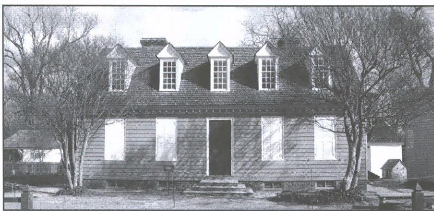
Brush-Everard house has been closed since the summer of 1994 for renovations. New climate control and security systems are being installed. The project was partially funded by a matching grant from the National Endowment for the Humanities. The house is scheduled to reopen Mon., April 17. Photo by Anita Hallman
