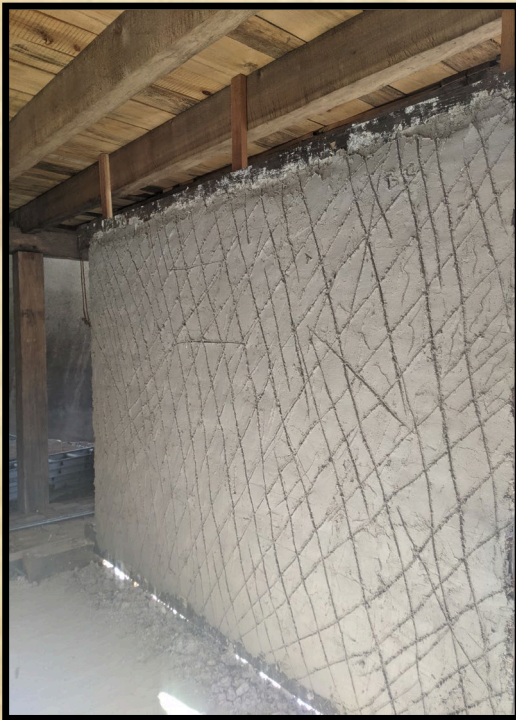
Scratch coat of the third practice wall.
