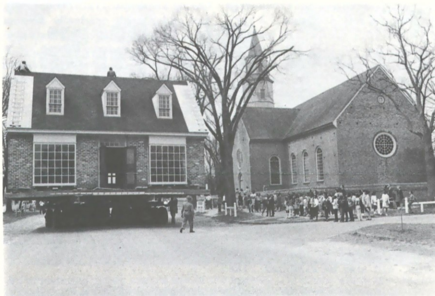
Above, the former Mr. Foster's Rememberance Shop near Bruton Parish Church on the Duke of Gloucester Street as it was being moved to its new location on the corner of Indian Springs Road and Jamestown Road.
