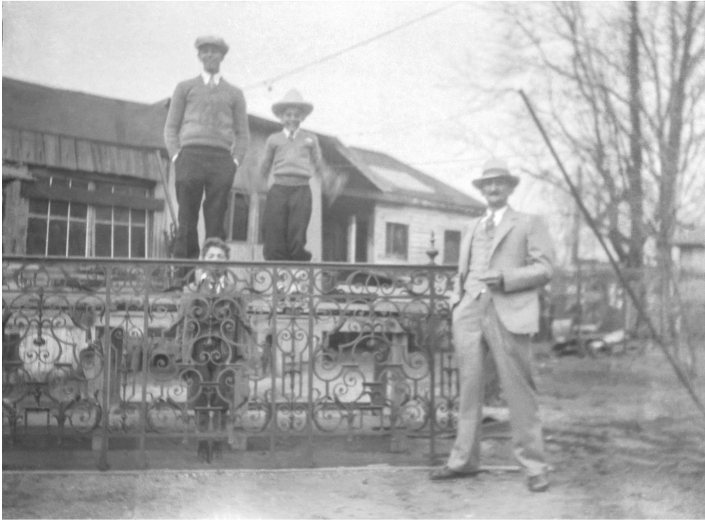
Governor's Palace balcony, completed. People are Ferrante "Fred" Ferrari, Ugo Tuccori, Fred Ferrari and Daniel Franceshi. Ferrante "Fred" Ferrari was an early contractor hired during the Restoration of Colonial Williamsburg.
