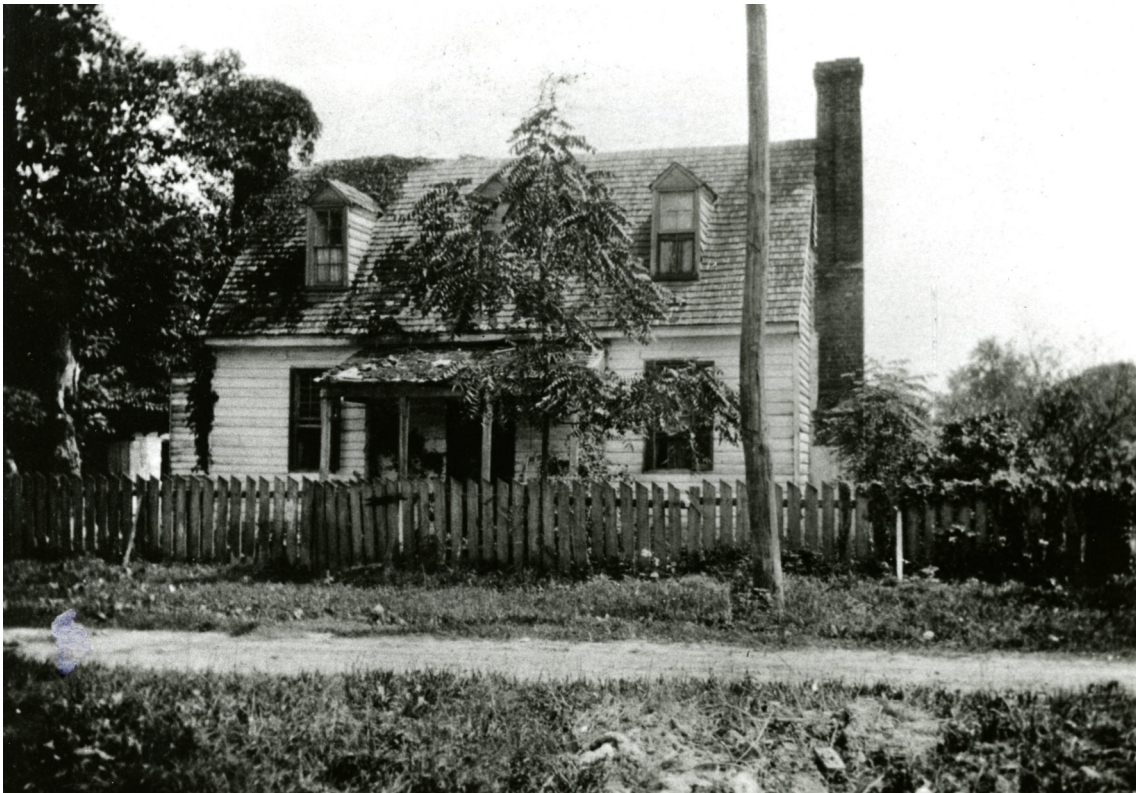
Front elevation of the Digges House, originally located on Block 23. Building 18 and moved to Block 24, Building 32, Williamsburg, Virginia.
