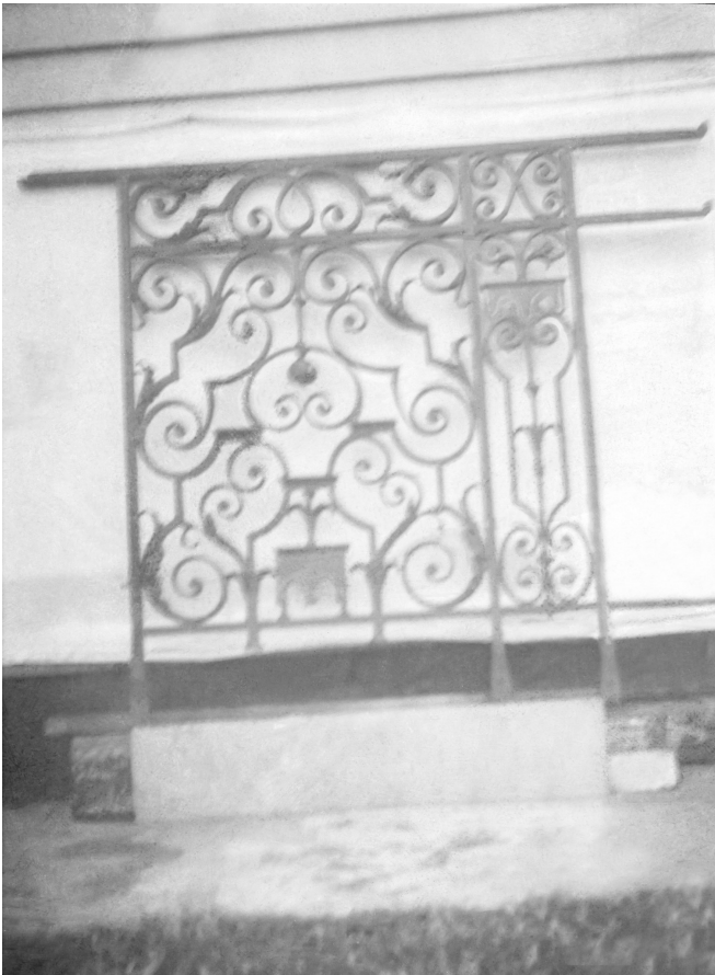
Governor's Palace balcony, in progress. Crafted by Ferrante "Fred" Ferrari, an early contractor hired during the Restoration of Colonial Williamsburg.
