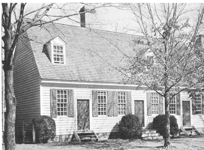
Reconstructed, the John Crump House looks once more as it did in Williamsburg's colonial days
