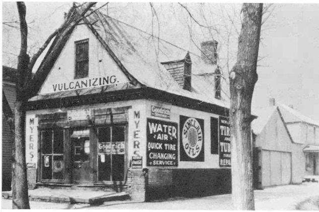
In the late twenties this eighteenth-century building was used as a garage
