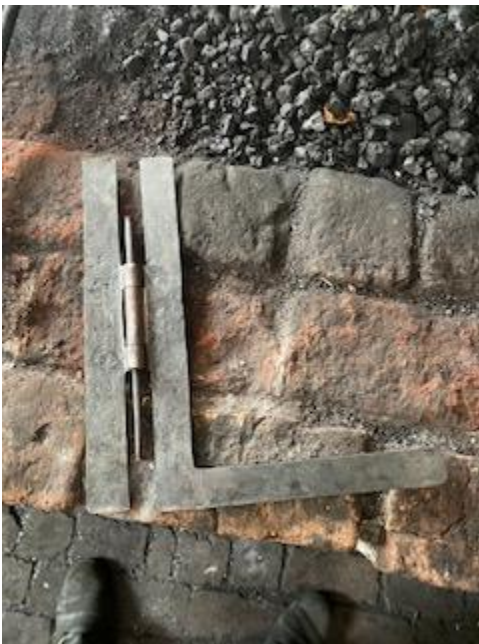
HL Hinge fit temporarily fit up with drift pin.
