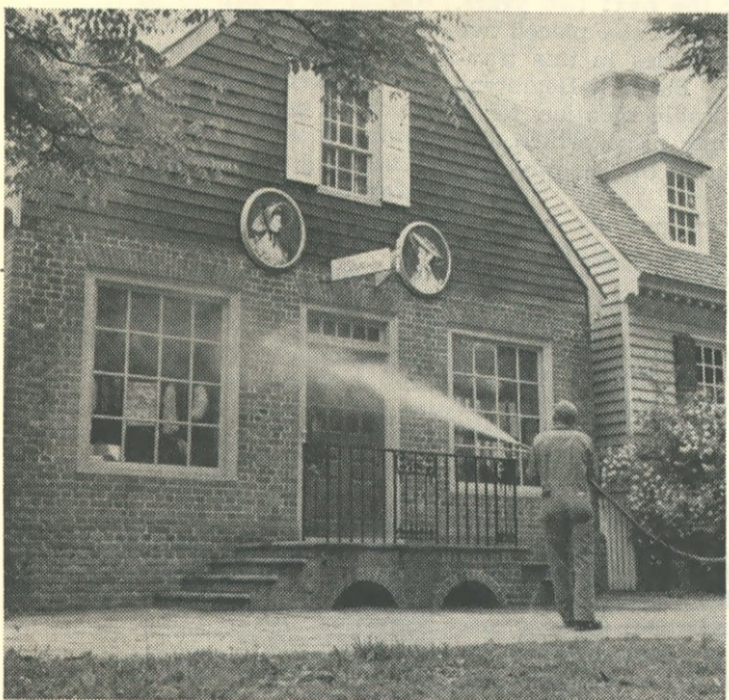
Buildings were also hosed down
