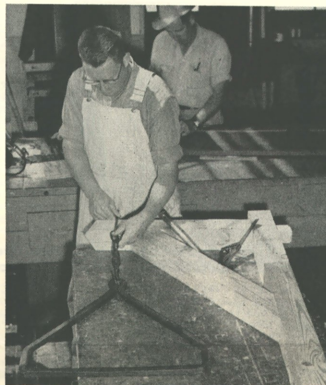
... carpenters made posts
