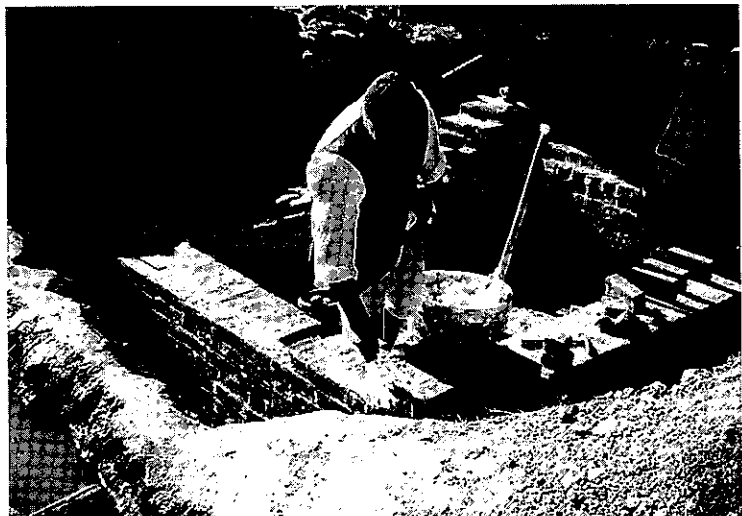
Figure 3. Working on the corner of the foundation of the north storehouse, Andrew Barry slides some mortar off his trowel.
