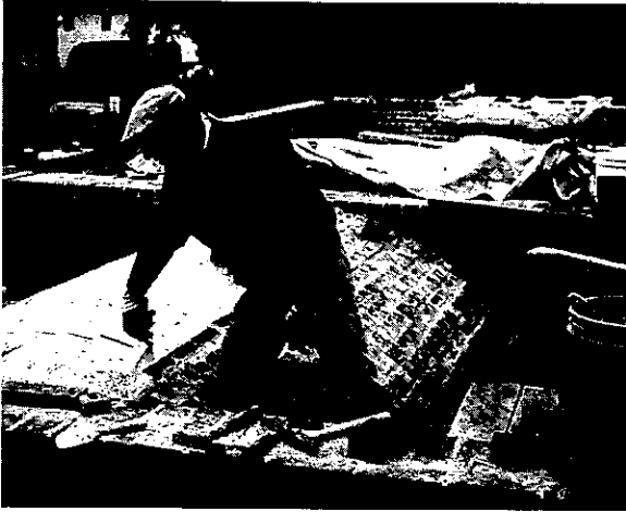
Figure 4. Raymond Cannetti lays a brick to the wooden form of the vaulted arch beneath the kitchen.
