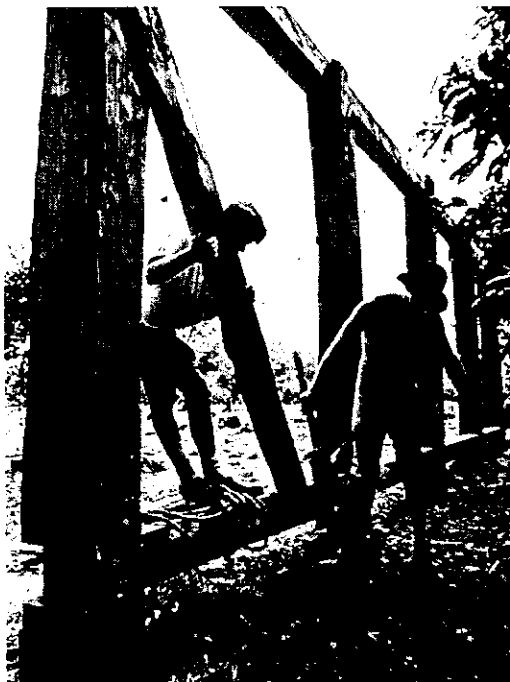
Great Hopes for Great Hopes: Housewrights are shown in the process of securing a wall during the raising of a building.
