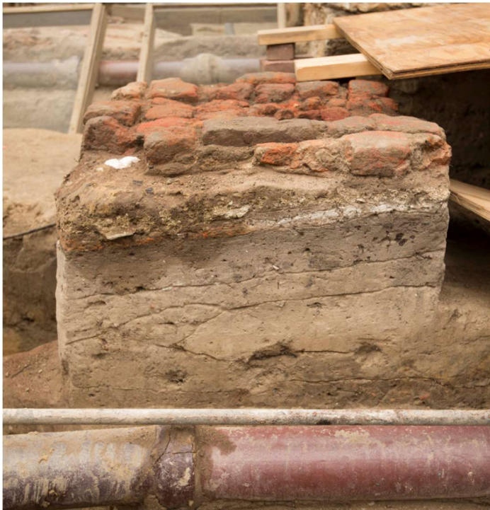
Figure 10: Brick paving above marl layer.
