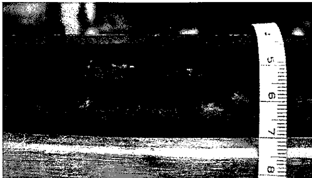
Linen pulley cord attached to lower window sash. Photo by Linda Baumgarten.
