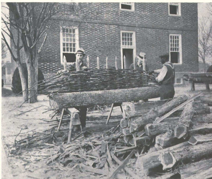
Illustrating how to make one of the most interesting fences now in Williamsburg. It is the wattle fence and can be seen at the Allen-Byrd House. The experts weaving one section of this picturesque barrier are S. D. Towler, J. S. Graves, and Calvin Jones, all of Construction and Maintenance.
