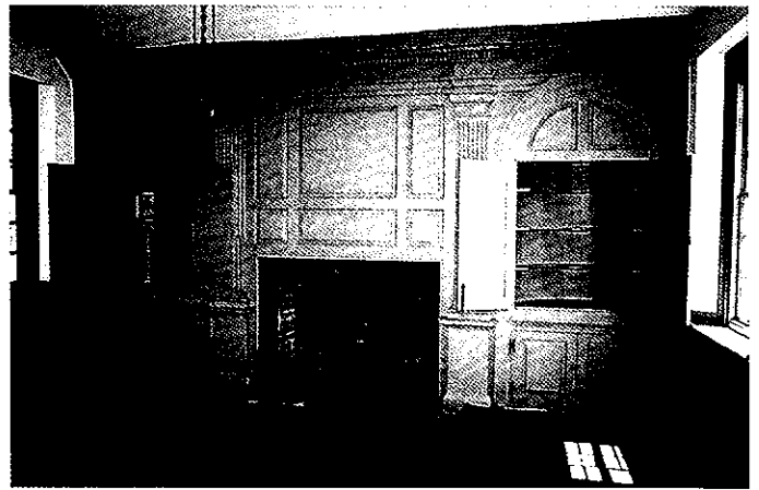
Hall, Smith's Fort, built circa 1763, illustrates the impressive paneling that could be found in dwellings of smaller but successful planters. Equipped with a pair of bowfats suitable for displaying and storing wares needed for meals and beverages, this room was the formal entertaining space for visitors who would have immediately recognized it as the most important room in the house.
