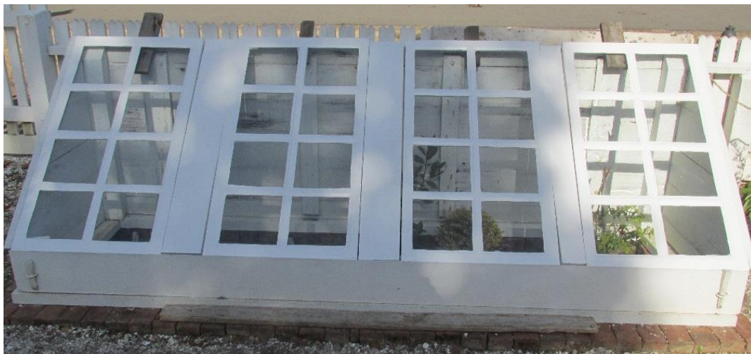
The freshly painted divided lights in place
