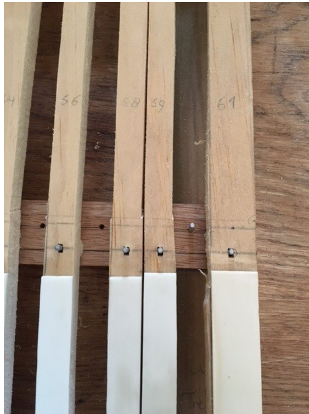
Balance Pins in New Key Pivot Holes.
