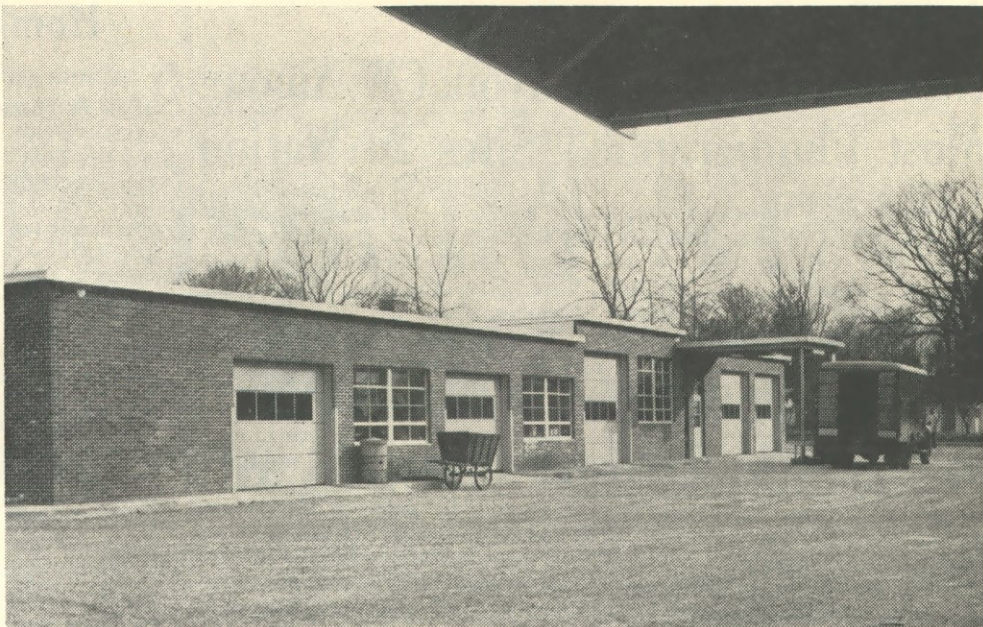
FIRST CLASS is the best word for the new Motor Shop. Here, one of CW's trucks gasses up at the service island. The new building provides improved facilities for general maintenance, overhaul, washing and waxing of the more than 70 vehicles owned by CW. The shop also maintains all landscape and construction motorized equipment.
