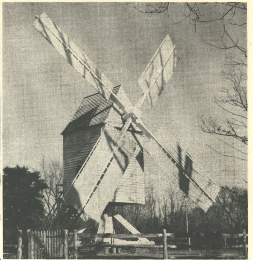
READY FOR THE BREEZE — Robertson's Windmill, currently nearing completion on North England Street, stands ready for a test run. Most structural work has been completed, and landscaping is in progress. Successful tests have already been made in grinding meal in the 18th-century fashion. When it opens to the public in late spring, it will be another free craft exhibit. Chiles Larson
