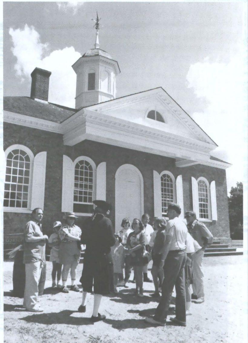
Before entering the court, visitors are "introduced" to the history of the 18th-century judicial system and the role of the Courthouse.
