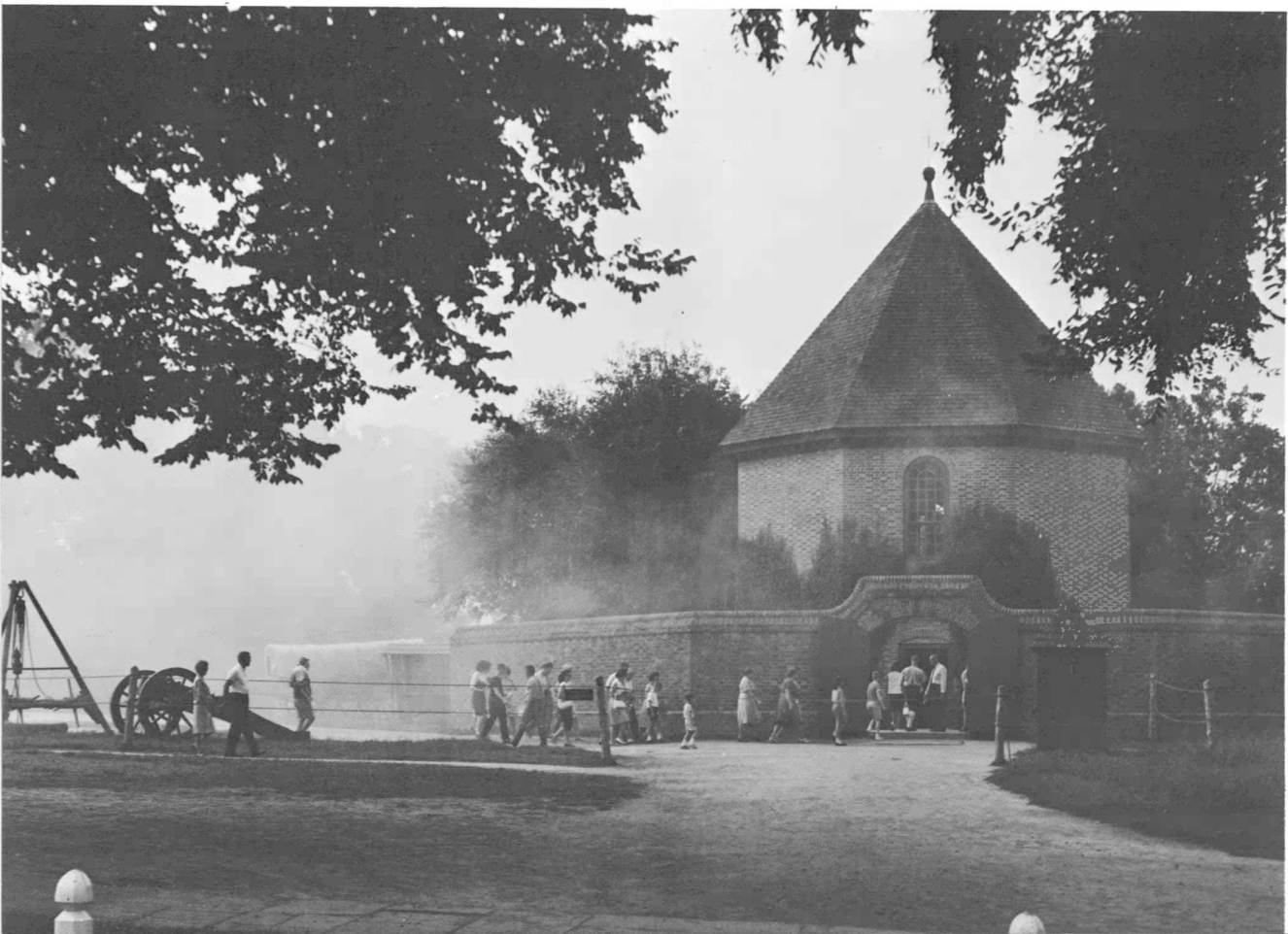
The restored Powder Magazine, most of its original masonry intact.
