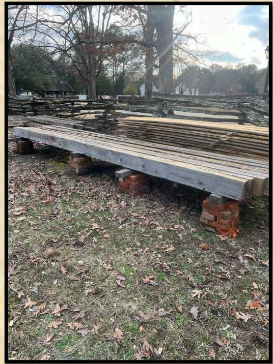
A newly stacked and stickered pile of framing.
