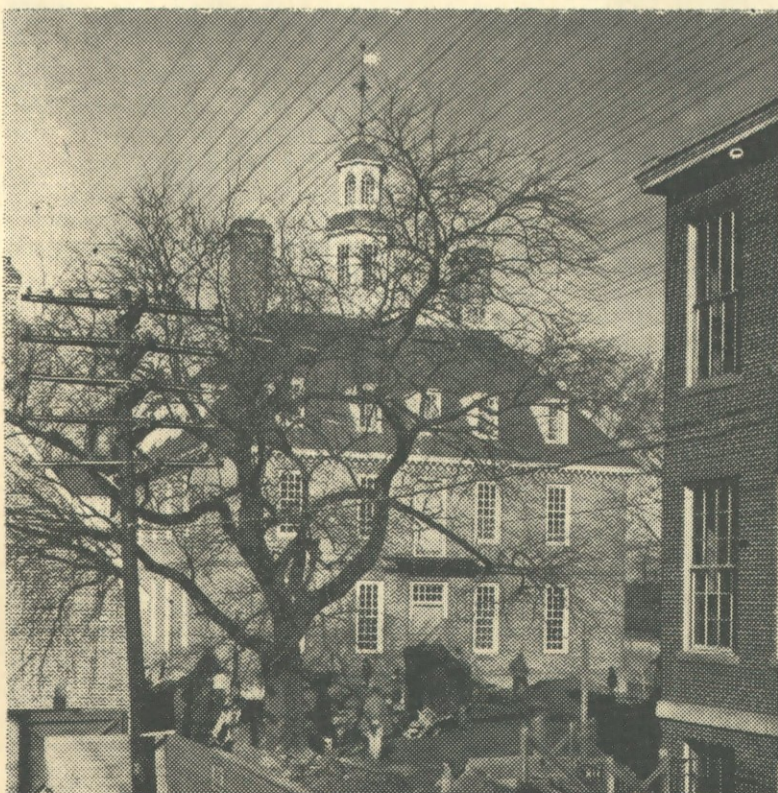
GOVERNOR'S PALACE was under construction on January 3, 1933 behind the old high school which stood at the north end of the Palace Green. Note overhead wires not yet removed.
