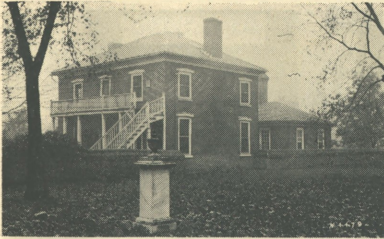
BRUTON PARISH HOUSE (the old one) provided office space for architects and builders before other facilities were available
