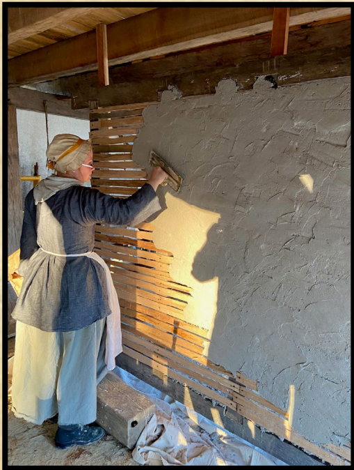
Madeleine applying the scratch coat
