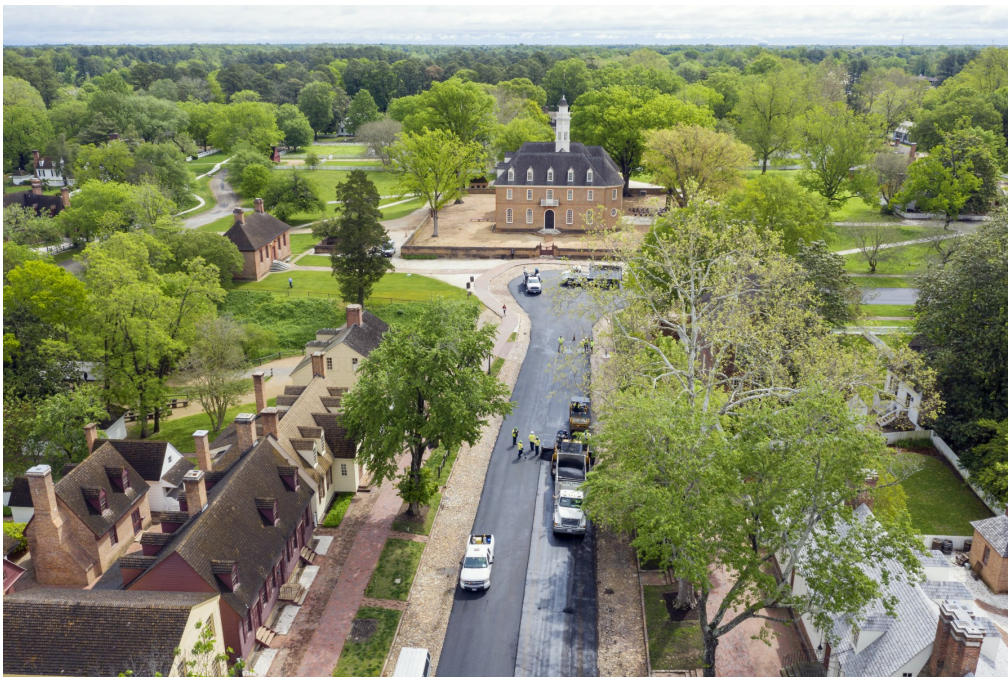
Duke of Gloucester Street repaving project
