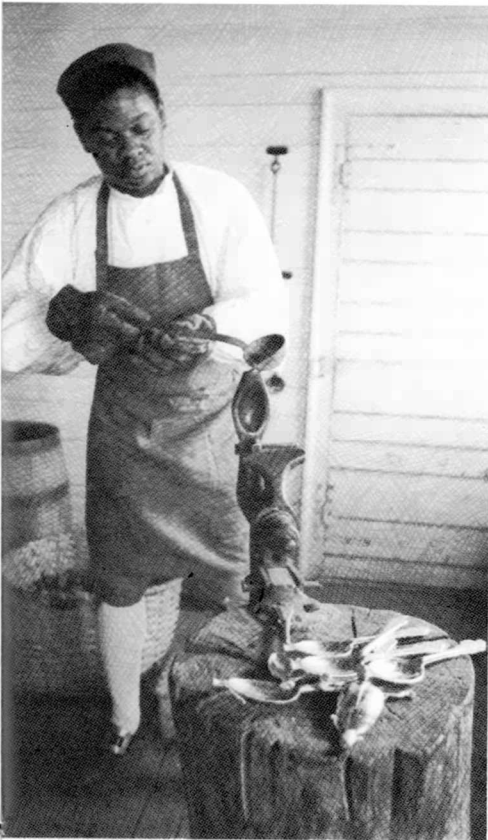
Pewter spoons come out of the molds by the hundred.
