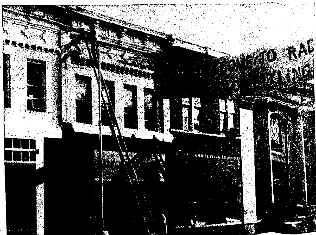
SOFT COLORS FOR HARD WARE — The Radford Hardware shop this week became the — er — umpteenth local building to join — uh — whatever that city beautifying project is called. Painters set up their ladders early Monday morning to
