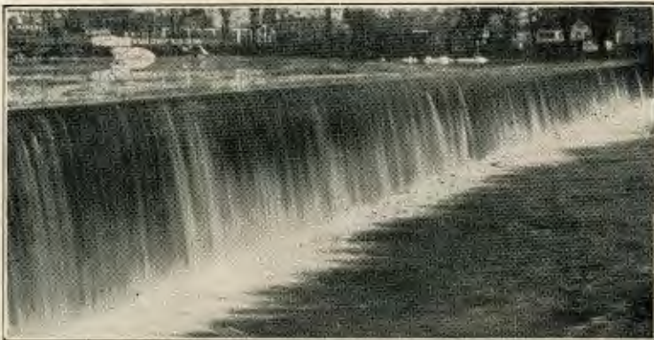
MERRIMACK RIVER DAM AT LAWRENCE
