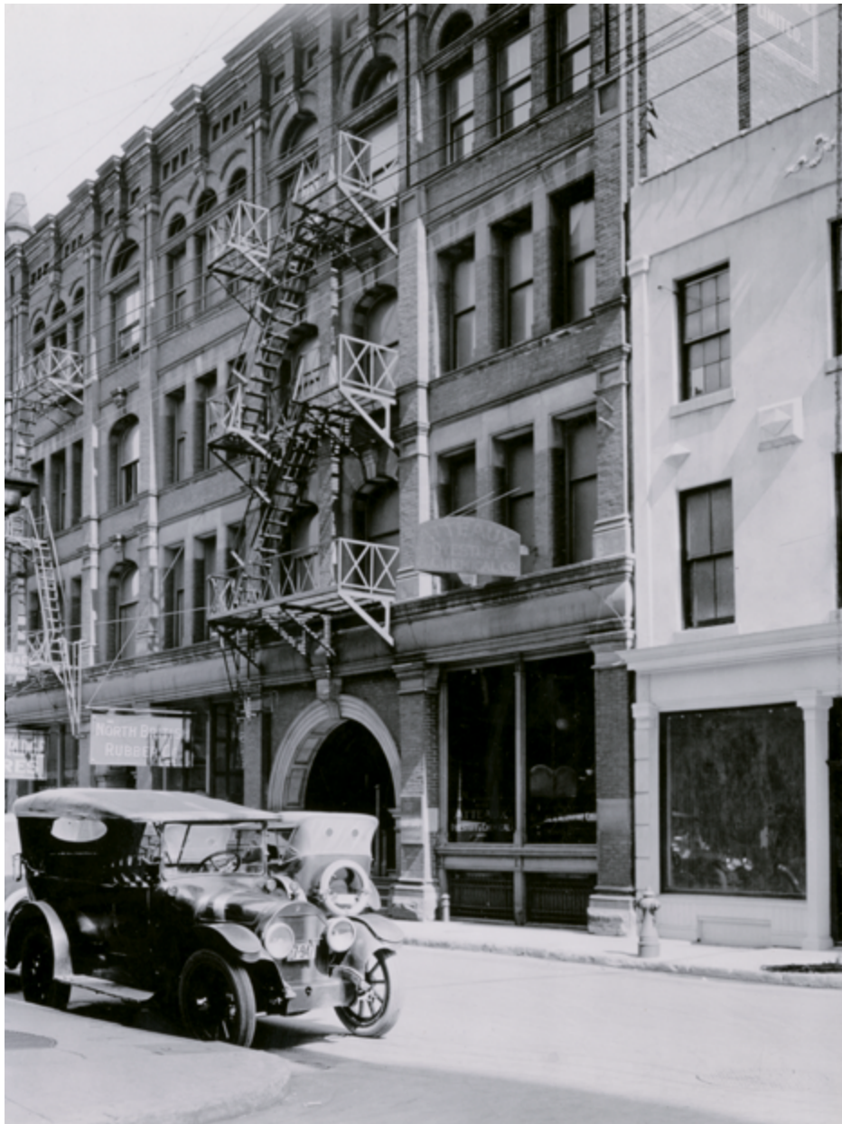
Canadian Kodak Co. [Canadian Kodak Co. building at 41 Colborne Street], ca. 1900 Gelatin silver print 22.9 x 16x5 cm
