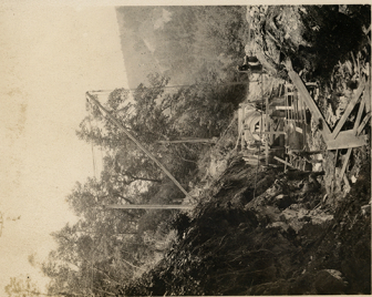
8' Concrete Pier Sta 414 S.W. RR. 7-27-06.
