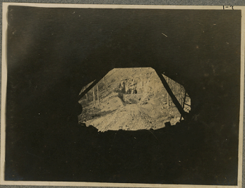
Speedy Tunnel from inside Pine Ridge
