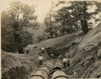
Uncovering broken Pipe Sta 394 - 48"
