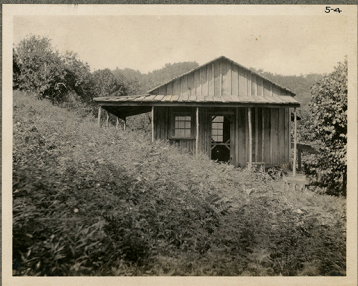
Division Engineer's Office - Camp #2 8-11-06
