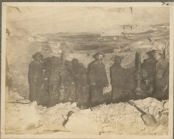
North Heading Lower Pine Ridge Tunnel - Camp #3 800 feet in. 4 air-drills at work.
