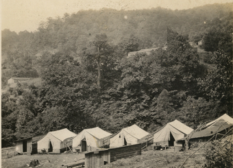
Moody & Glenn Concrete Camp - Camp e S & W.
