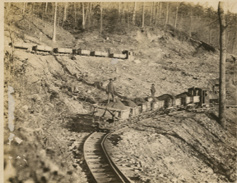
7-1 Dirt Trains Shovel No 8 54000 cubic yard Cut Station 418 Camp No 2 S & W R.R.
