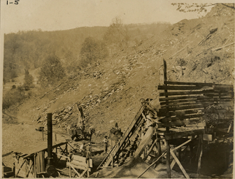
Rock Crusher 8' x 10' Culverts Camp #2
