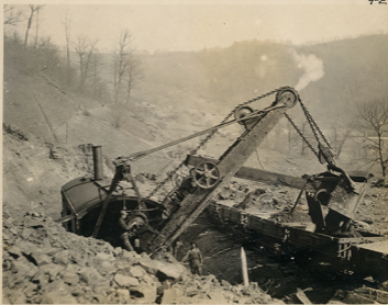
Model 60 Shovel working in cut near Camp #2 3-22-07
