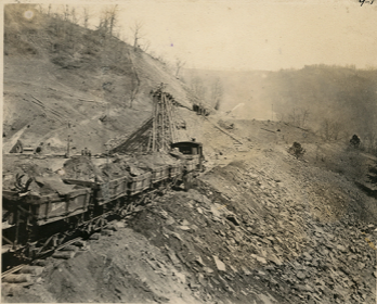
Making 175,000 Fill near Camp #2 S2 W.R.R. Altapass, NC 3-22-07
