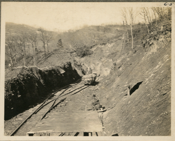
Steam shovel N88 working against breast 83 ft deep Camp No 2 S. & W. RR. Well-drill on top. 11-16-06
