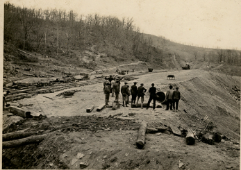
Pulling 48 inch pipe up embankment (100') with Locomotive 75 4-1908 Alfred, N.C.
