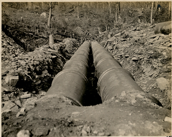
Double line 48 inch Cast Iron Pipe Camp 2 L.C. path 252 feet. May 07.
