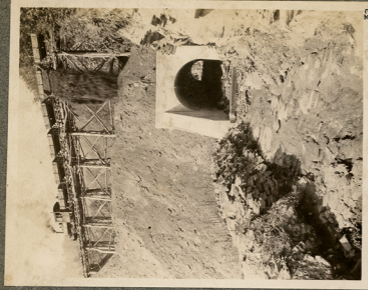
Covering 10 ft Arch Culvert Camp 2 S.E.W. R.R.
