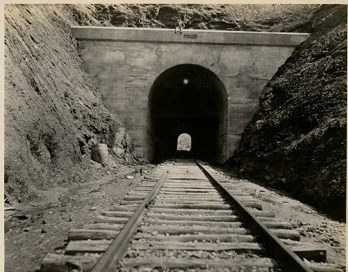
North Portal Vance Tunnel - Allapass, N.C. 9-29-07. Hathorn S.E. W. RR.
