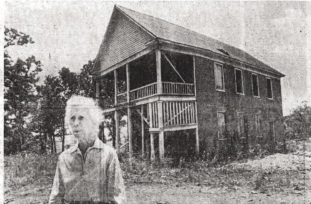
Jane Armstrong stands in front of the old Maxwell Academy building, where she went to school and later taught. New Providence Presbyterian Church once operated the school.
