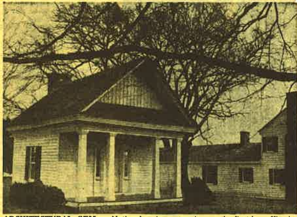
ARCHITECTURAL GEM — National Park Service experts have termed Landon Carter Haynes' law office a perfect example of Greek Revival architecture. This small building, recently restored, was the first law office in what is now Johnson City, and Haynes was the town's first lawyer. So important was he that the settlement was then known as Haynesville.
