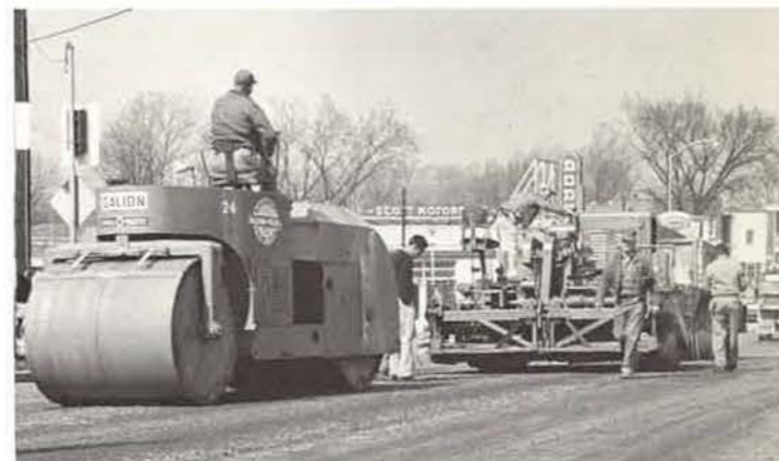
493 tons of asphalt used in 1960-61 for repair of paved streets.
