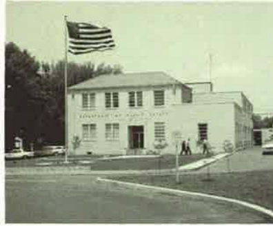
Your new Public Safety Building, with its attendant functional aspects and morale factor, is a noteworthy addition to the City.
