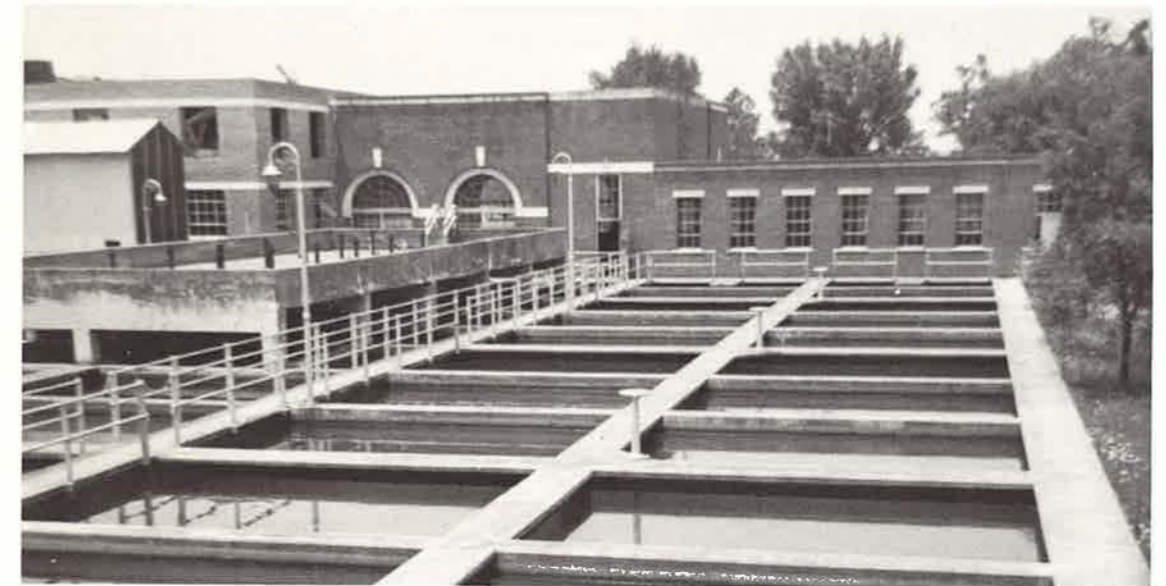
WE ANTICIPATE YOUR NEEDS: The present Filter Plant has a daily filtering capacity of about 6,000,000 gallons and, when this addition is completed, will have a capacity of 8,000,000 to 10,000,000 gallons of water daily.
