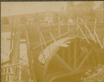
Forms for 25' Concrete Arch - 15° skew over Little Tondaway Creek
