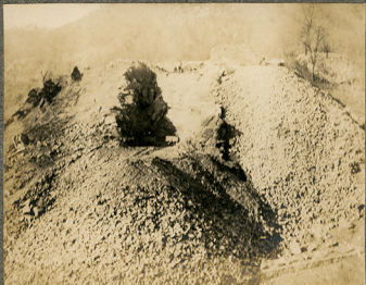
To cut Sta 720 Wasting Top Lift
