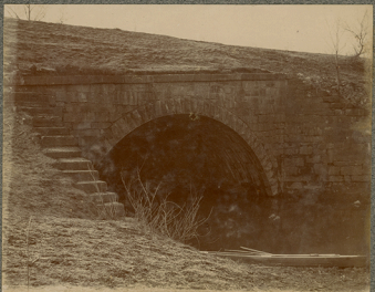
Little Tonoloway Aqueduct C&O Canal Hancock Md.
