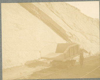
Cut Sta 620 Showing Rock Slope
