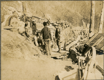
Smith Mixer - Retaining Wall Sta. 755
