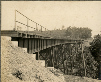
Steel Viaduct at McCoys Ferry W.M.R.R.
