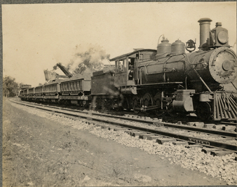
Borrow-pit Ft. Frederick Md. Gaton Shovel. W.M.R.R.
