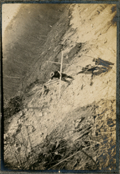
Difficult cross-sectioning Sta 755
