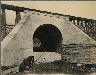
15' Roadway Culvert Near Clear Spring Md. W.M.R.R.
