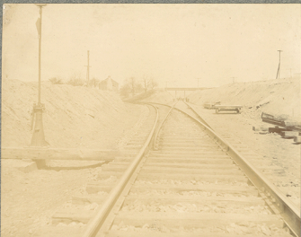
Where Cumberland Extension Left Main Line WM R.R. Big Pool
