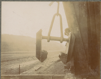
Clamps for Lifting 25 ton Girders
