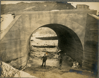
25'-15" Skew Concrete Arch Little Tanoloway Creek
