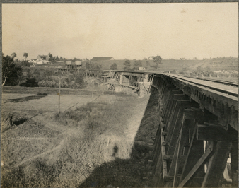
Conococheague Bridge & Trestle W.M.R.R.
