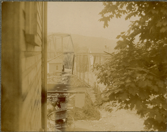
Canal & River Bridges Hancock Md Town "Jail"
