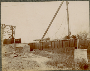
Tonaloway Girders in process of erection
