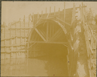
25' Concrete Arch Forms Little Tondaway
