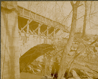
Great Tonnolaway Aqueduct C & O Canal
