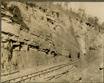
Rock Cut Dam No 6
