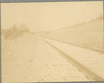
New Track - Wagon Bridge
