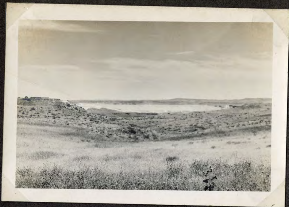
Enders Dam under construction 8-11-49
