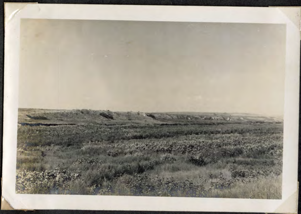
Looking West - note steep shoreline 7-27-49
