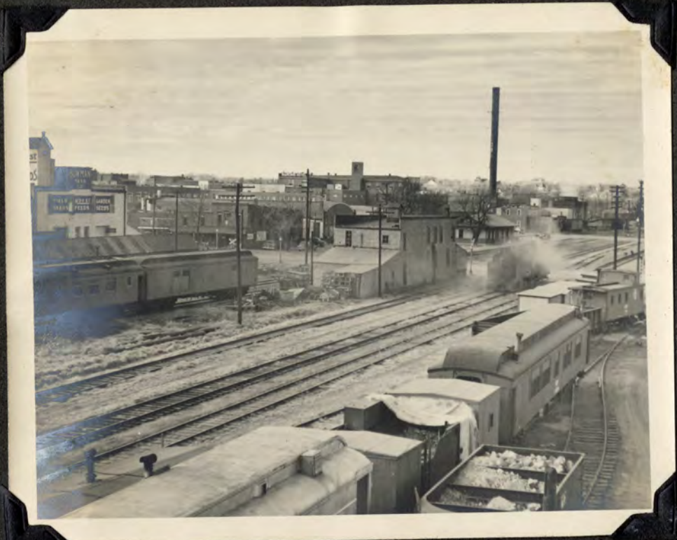
From Viaduct looking SW over RR 11-29-49
