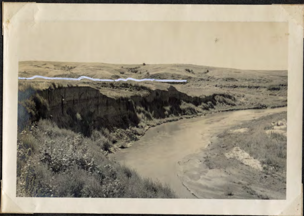
Central Basin - note rolling hills and approx. Normal Pool Contour 7-27-47
