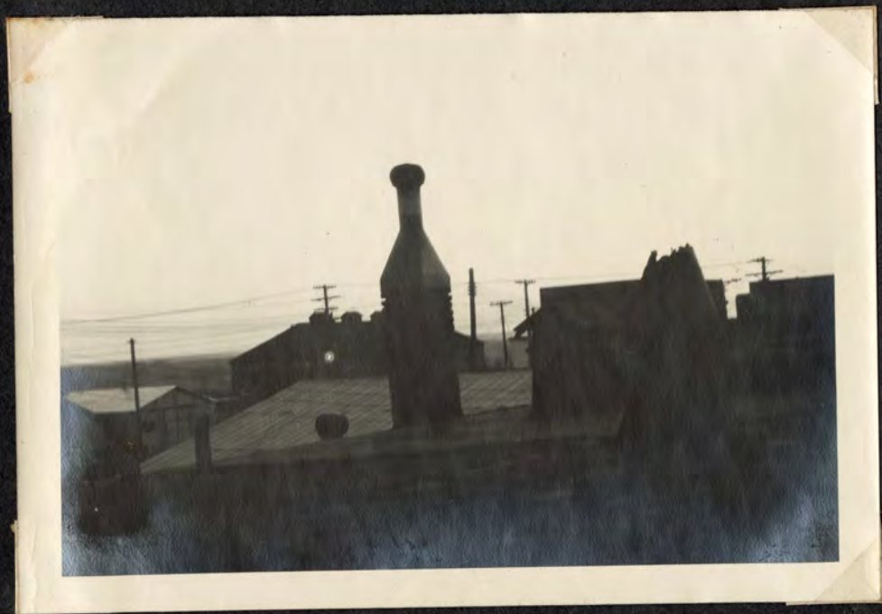
Roof tops - McCook, Neb
