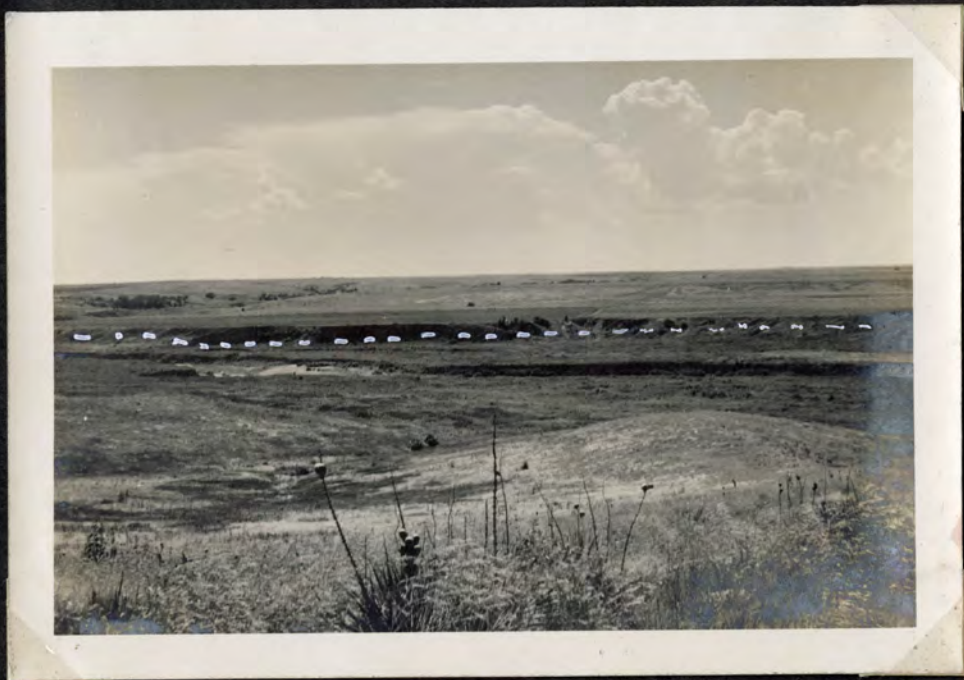
Steep shoreline near upper end of Contour 7-28-49
