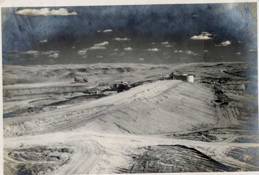
Enders Dam - under construction 8-4-49
