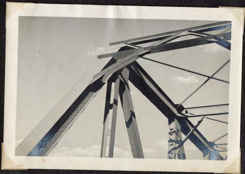
Bridges near Orleans, Neb.
