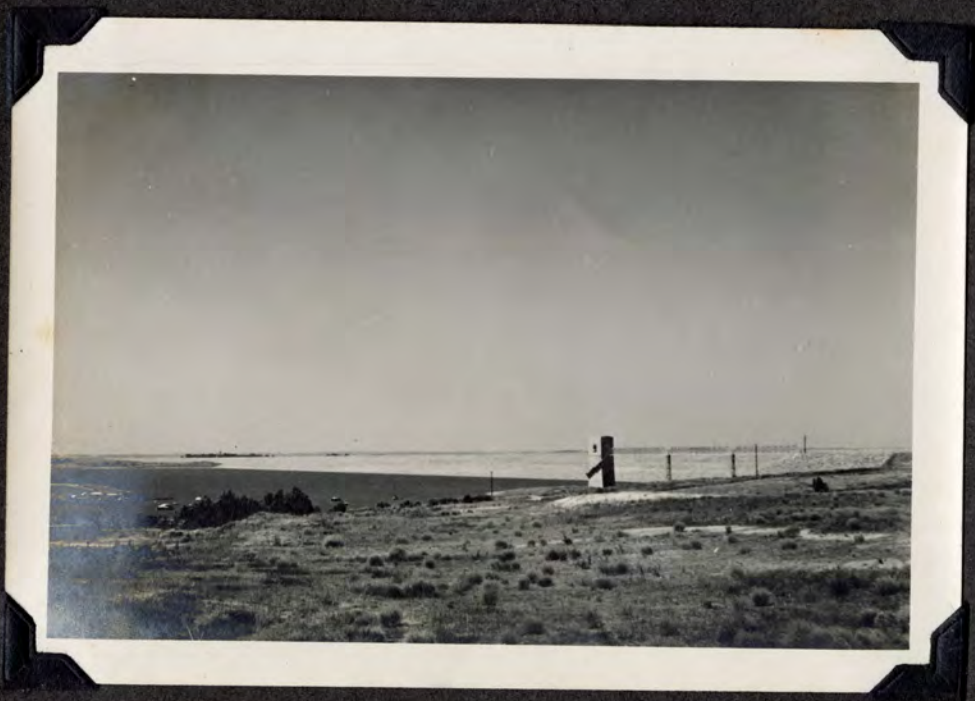
Kanopolis Dam, June 30, 1949
