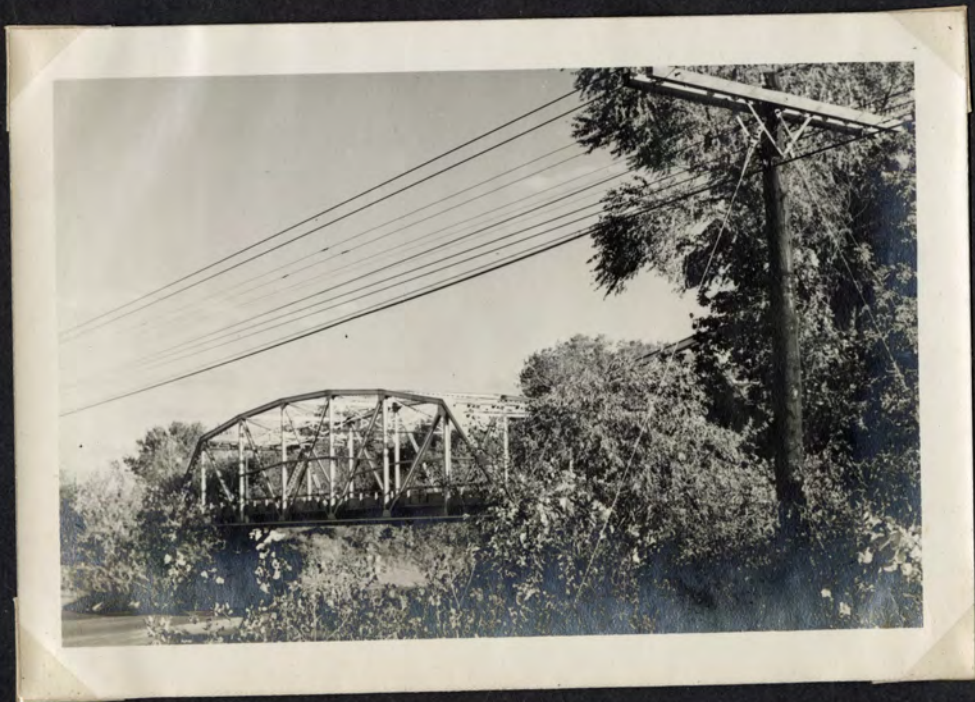
Bridges near Orleans, Neb.
