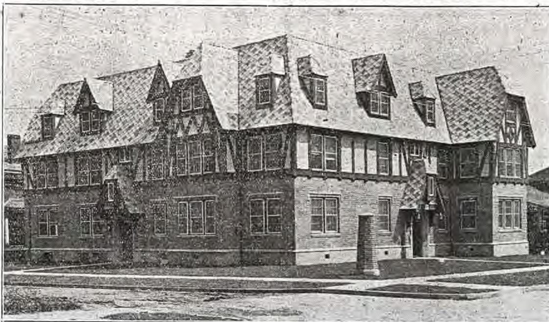
One of the most handsome structures of the city is the Wex-Jo-Leon Manor, completed last August. It is located on Broad and Ravine Streets with main entrances on either street.
