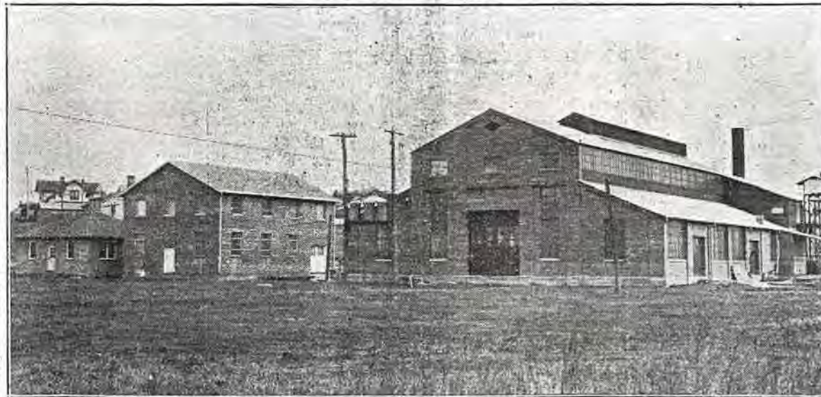
Plant of the Kingsport Foundry and Manufacturing Corporation. The large building to the right and in the foreground is the foundry and machine works building. To the left and rear of it is the pattern shop building and pattern storage room. The building to the extreme left and in the background houses the offices.
