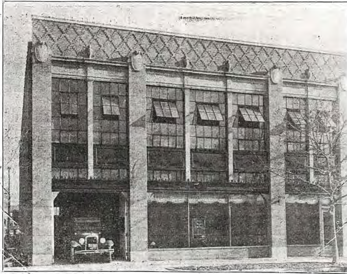
Handsome home of the Chevrolet, located at Center and Cherokee streets, showing front entrance on Cherokee. Cars are given splendid display in the spacious show room.
