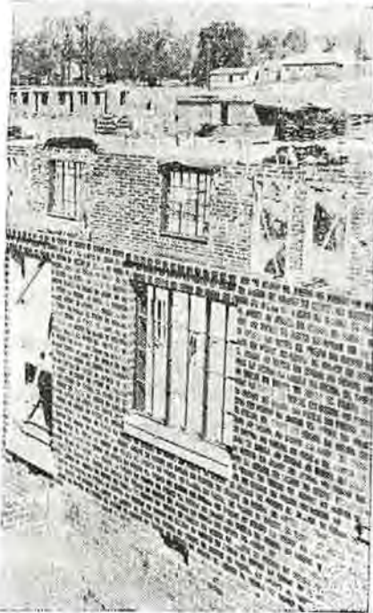
Kingsport's low-rent housing projects are rapidly taking shape as revealed by the pictures shown here. The project for white residents, upper left, now is 25 per cent completed and will house 128 families in 20 buildings. The pictures above and at right show the construction of the project to house 48 families of colored residents six buildings scheduled to be completed by August 15. When both projects are completed a maximum of 204 houses in the slum areas of the city classed as sub-standard will be razed. Each of the buildings is of brick and concrete construction and fireproof throughout. Construction was made possible through a loan-grant from the United States Housing Authority to the Kingsport Housing Authority which matures within 60 years.
