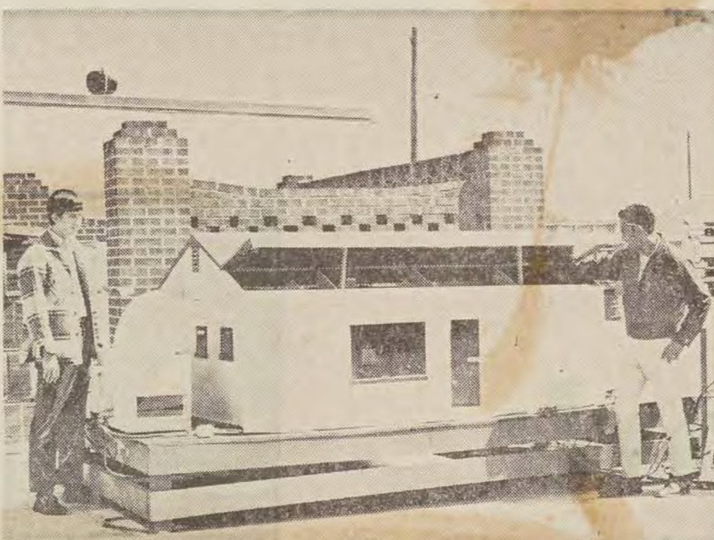
SPECIAL PROJECT — A model home, complete with heating and air conditioning, fully automatic seasonal changeover, was designed by the air conditioning engineering technology class at F. T. I. and built by students in the air conditioning trade group. (Photo by Payne).
