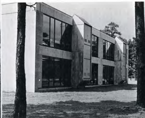
An angle view of the front of the new building.
