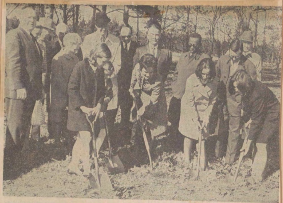
GROUNDBREAKING—Groundbreaking ceremonies were held for the Paul H. Thompson Library at Fayetteville Technical Institute Thursday morning. Members of the board of trustees, the faculty, staff and student body watch as Mrs. Thompson (center)
