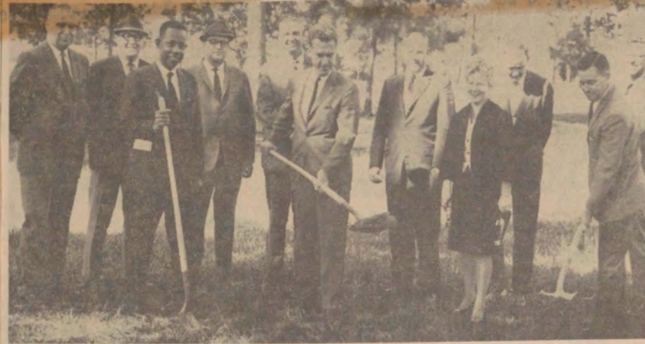
GROUND BREAKING — Members of the board of trustees of Fayetteville Technical Institute broke ground Tuesday for a new eight-classroom building, the first building to go on the Institute's new 48-acre campus expansion. From left are William West, E. L. Cameron, Jr., president, DWC Con-
