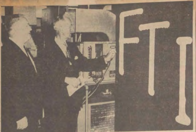
DECKER TOURS FTI — Alonzo G. Decker Jr., president of Black and Decker Manufacturing Company, toured Fayetteville Technical Institute Wednesday afternoon. Here Decker examines a display of frost covered pipes reading FTI in the school's air conditioning and refrigeration classroom. Howard Boudreau, left, president of FTI, conducted the tour. Decker was principal speaker at the graduation exercises. (Observer photo—Shaw)
