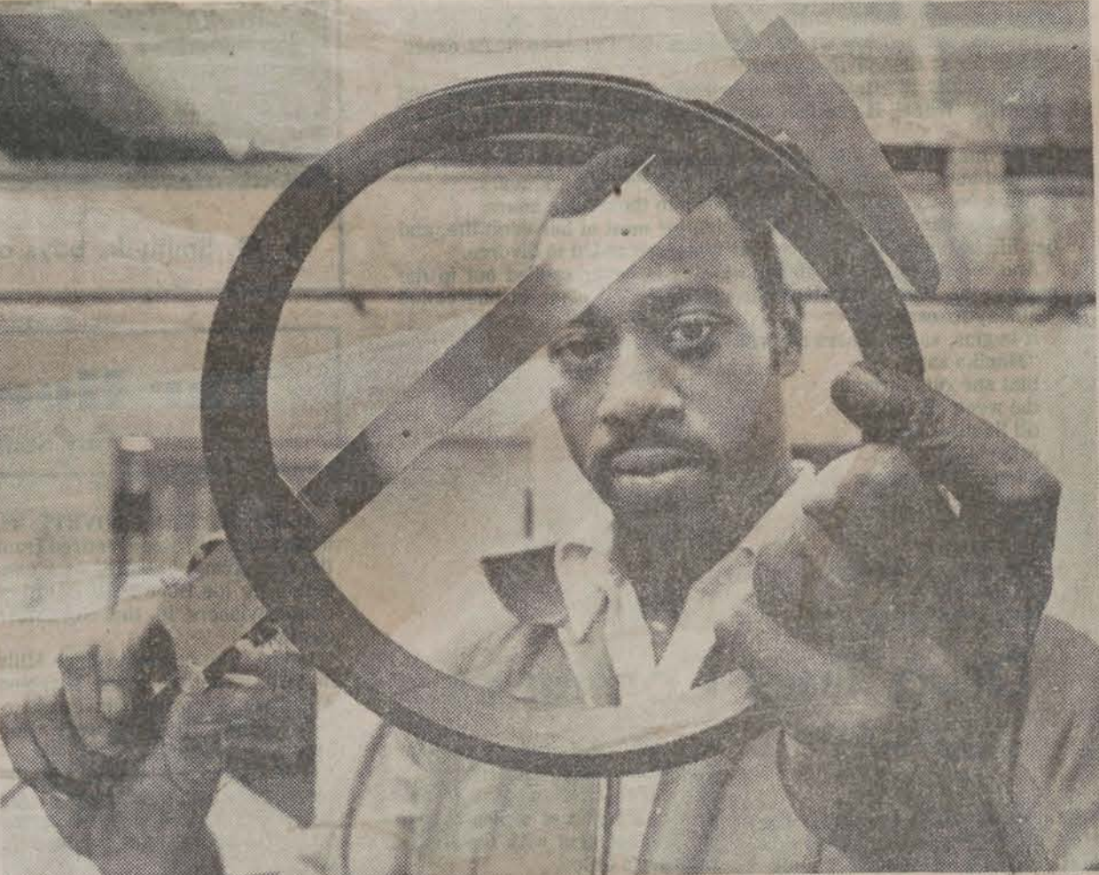
Andrea Lilly uses calipers to check measurement of a pump seal
