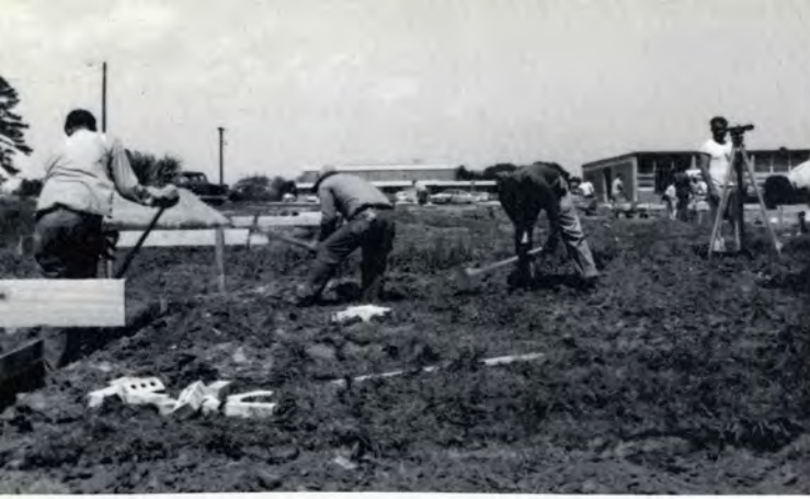
Breaking Ground and Layout of Foundation
