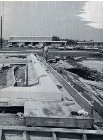
Fabrication of Pre-stressed Reinforced Concrete Beams at the Construction Site
