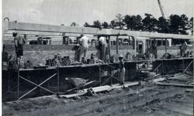
The walls go up on the West End Addition.
