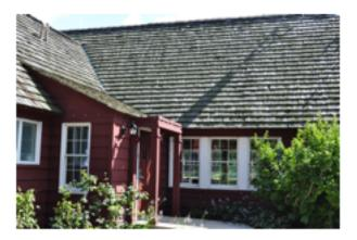
The 1959 addition to the building extends the footprint of the building to the south. The change in roofline clearly delineates where the original 1937 building ends and the 1959 additions starts. The 1959 plans show an overhead door on the south side of the addition, extending almost the full width of this part of the building.
