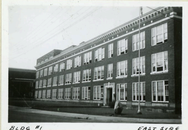
BLDG #1 EAST SIDE
