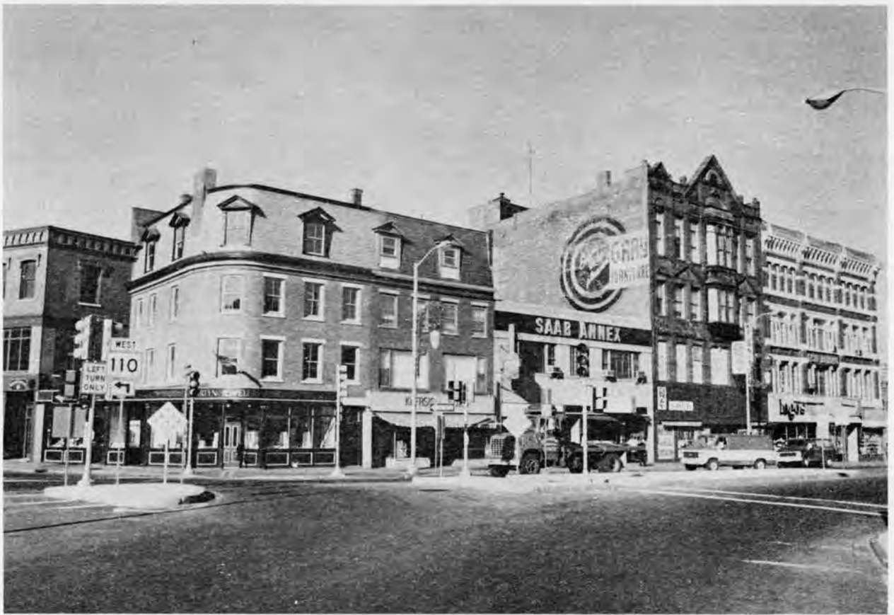
Figure 4-17 View of the Central Street block between Middlesex and Jackson Streets, 1979.
