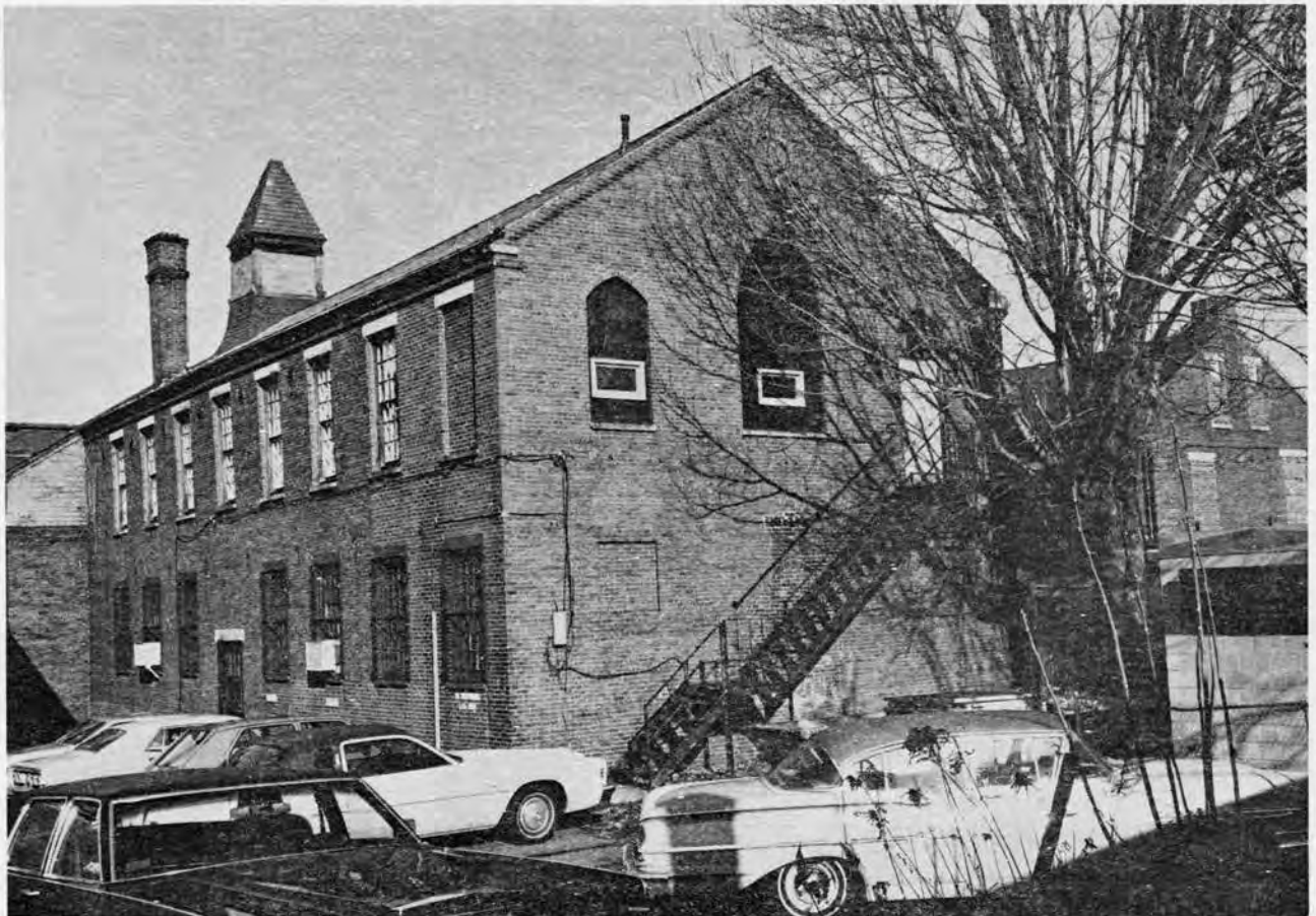
Figure 4-23 Rear view of the Free Chapel and the Elliot School.
