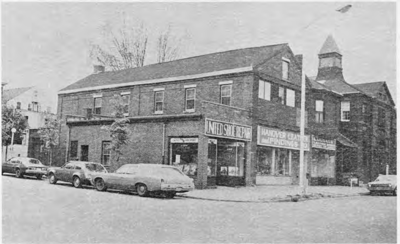
Figure 4-22 View of 140 Middlesex Street (the Elliot School, center) and 150 Middlesex Street (the Free Chapel, right) from the northeast.
