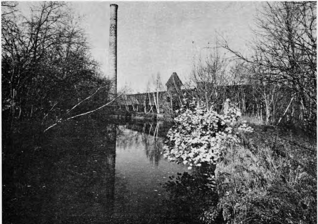
Figure 4-25 View of the Wamesit Canal behind Stirling Mills, 1979.
