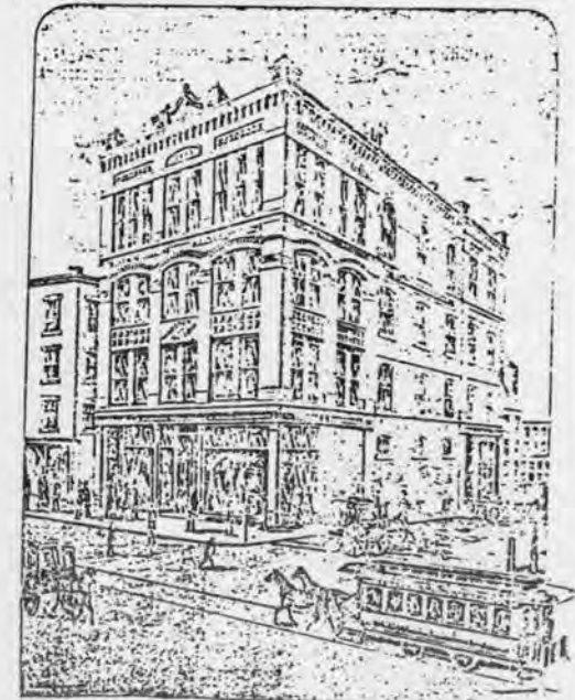
THE MARSTON BUILDING, MIDDLESEX STREET
