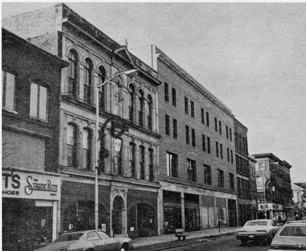
Figure 3-29 View along Merrimack Street, 1979.
