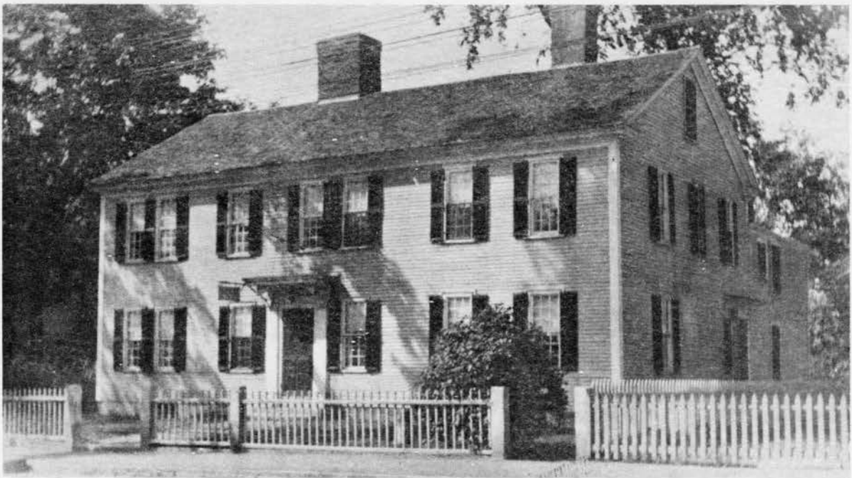
Figure 3-2 Spalding House, 383 Pawtucket Street, built 1761, photographed ca. 1920.
