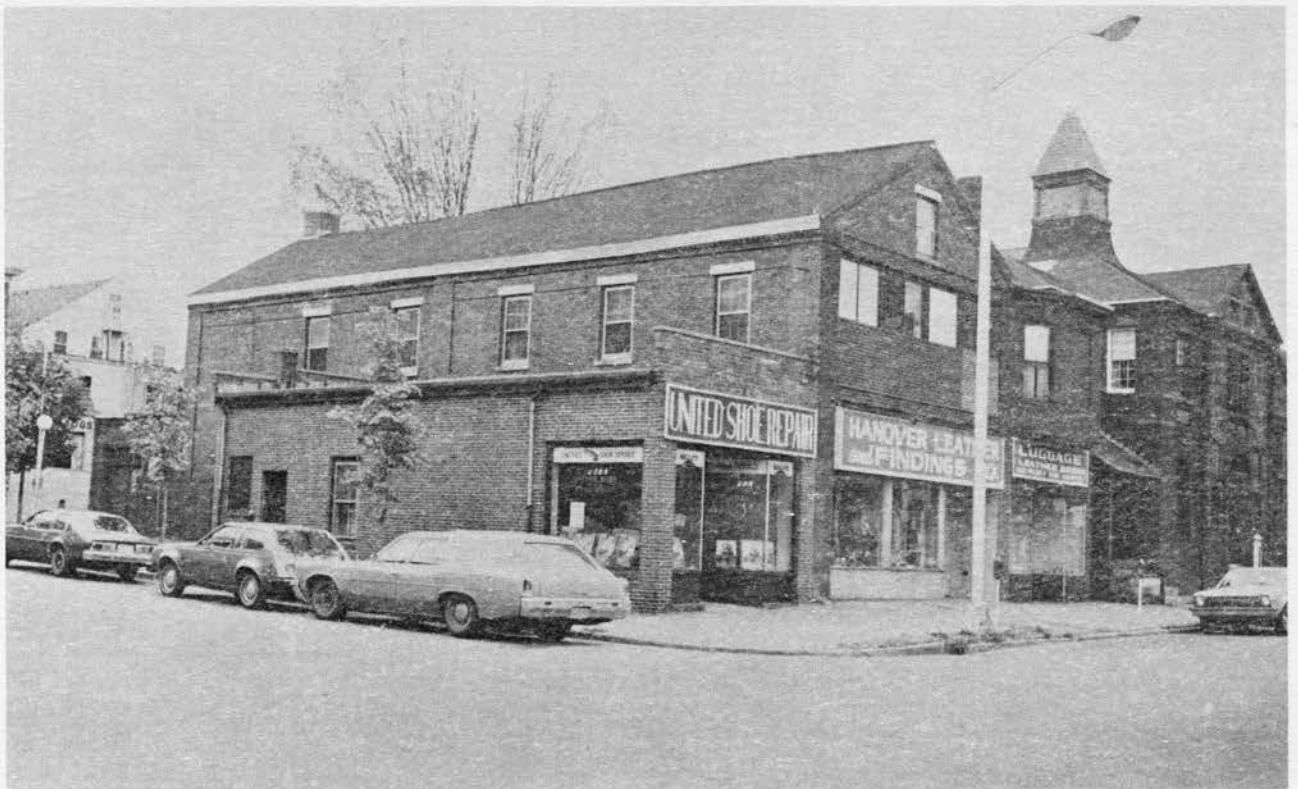
Figure 4-22 View of 140 Middlesex Street (the Elliot School, center) and 150 Middlesex Street (the Free Chapel, right) from the northeast.
