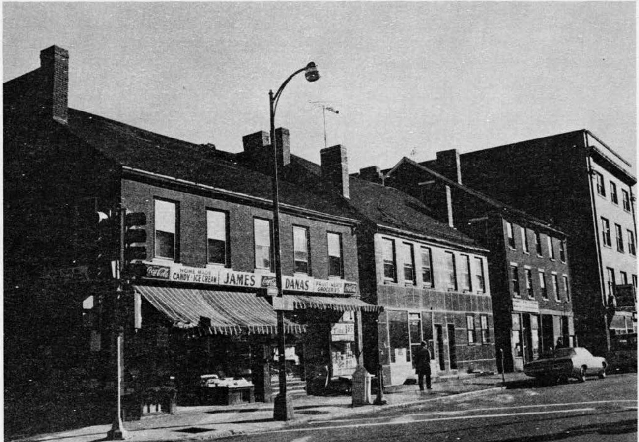
Figure 4-19 View of 62, 72, and 80 Gorham Street (left to right), all built ca. 1830, photographed 1979.
