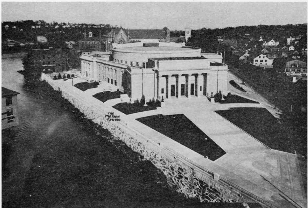
Figure 3-36 Lowell Memorial Auditorium, as it appeared when built in 1923.
