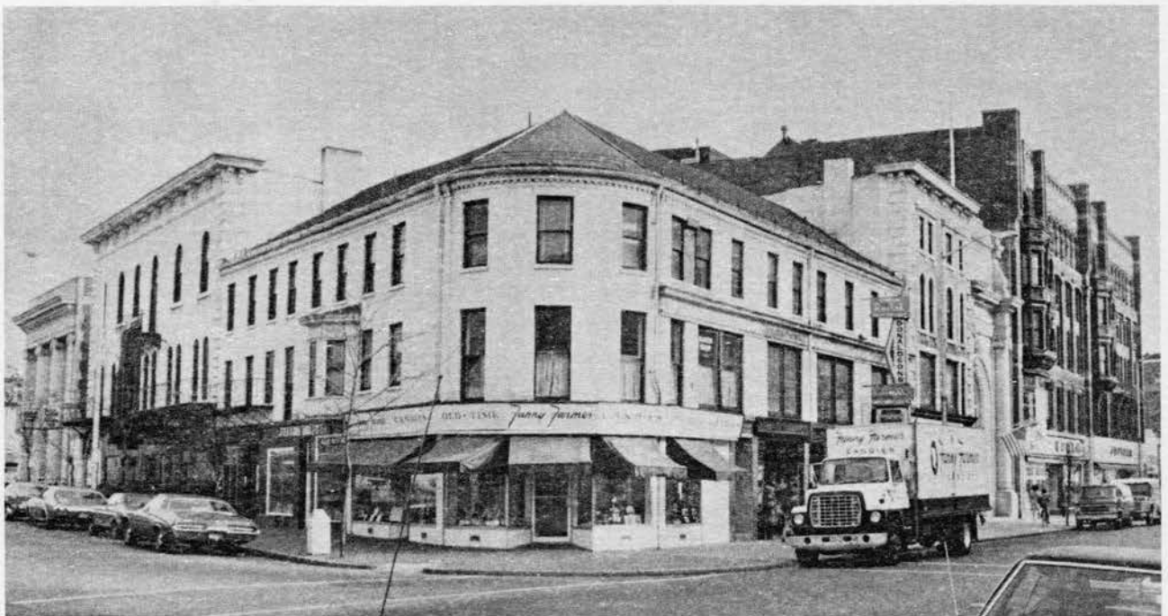
Figure 4-4 View of the Nesmith Buildings at the corner of John (left) and Merrimack (right) Streets, 1979.
