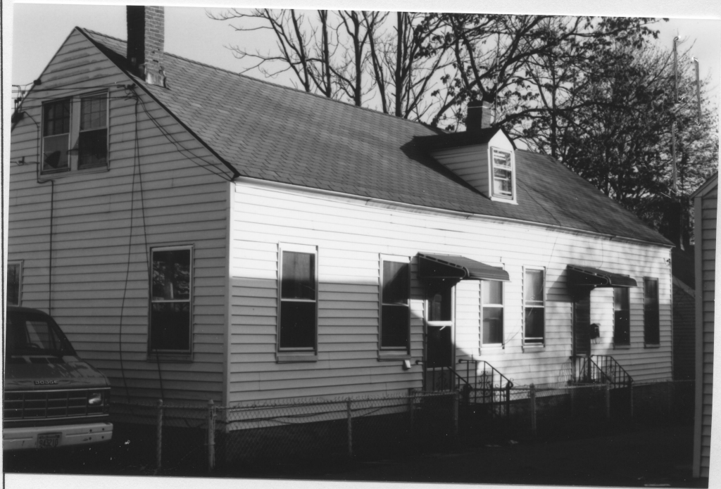
VIEW FROM northwest PHOTO TAKEN Nov.1992
