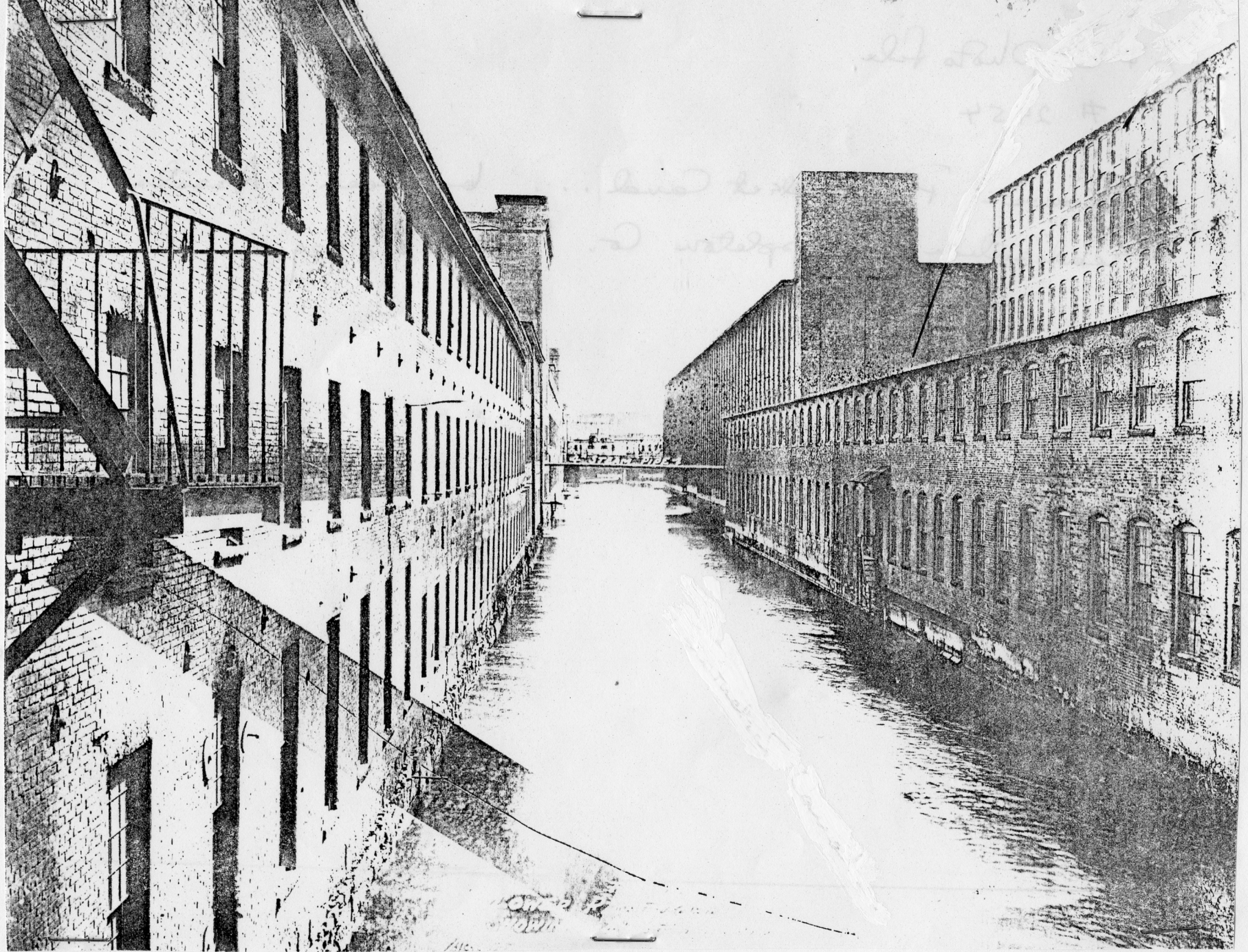
View from the west along the Pawtucket Canal, 1929. The Appleton Dye House is at right. U. of Lowell Library, Special Collections, Locks and Canals photo #2454.
