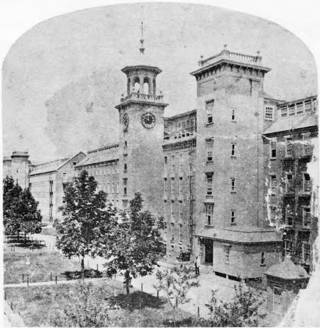
Figure 3-20 View from the southeast in the Boott millyard, ca. 1870.
