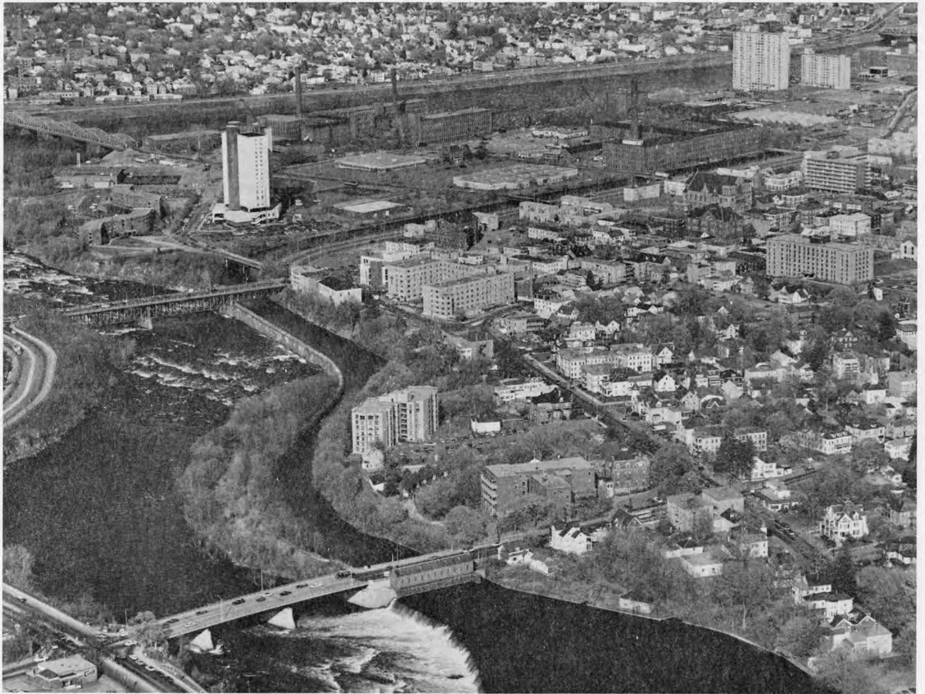
Figure 3-17 Aerial view of the Northern Canal, 1979.
