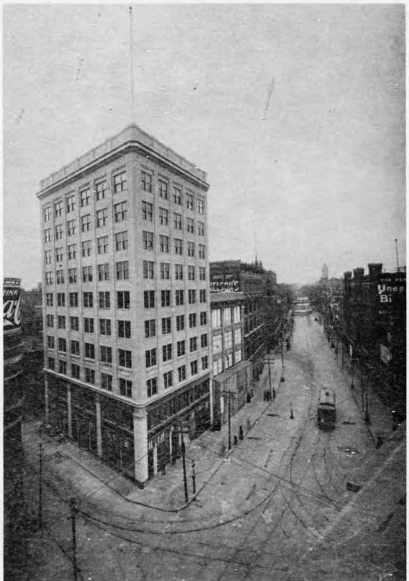
Figure 3-35 Lowell Sun Building, as it appeared when built in 1910.
