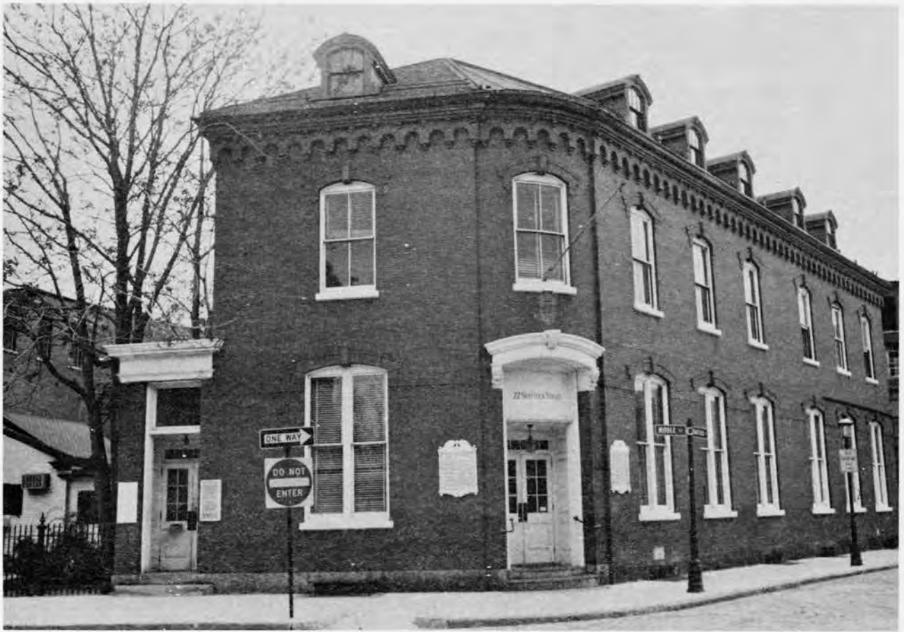
Figure 3-21 Lowell Gas Light Company, 22 Shattuck Street, offices of the Lowell Historic Preservation District Commission. Built 1859, photographed 1979.
