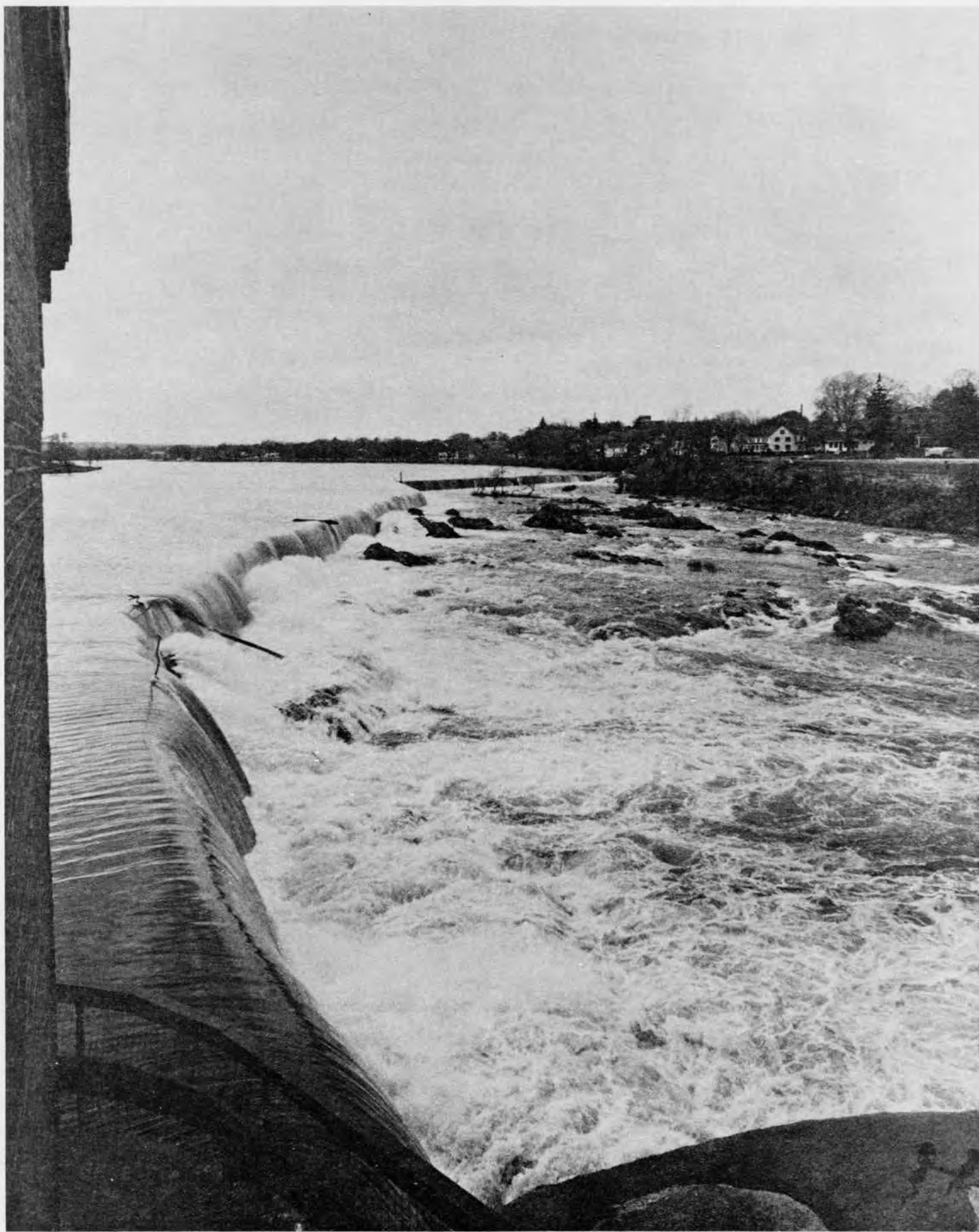
View of the Pawtucket Dam and Falls from the northeast, 1979.
